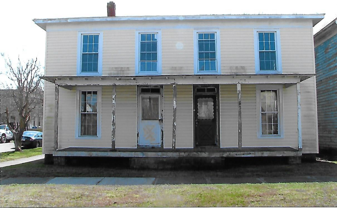
EXISTING FRONT ( NORTH ) FROM RANDOLPH AVENUE ( INCLUDING EXISTING PORCH AND STEPS )
