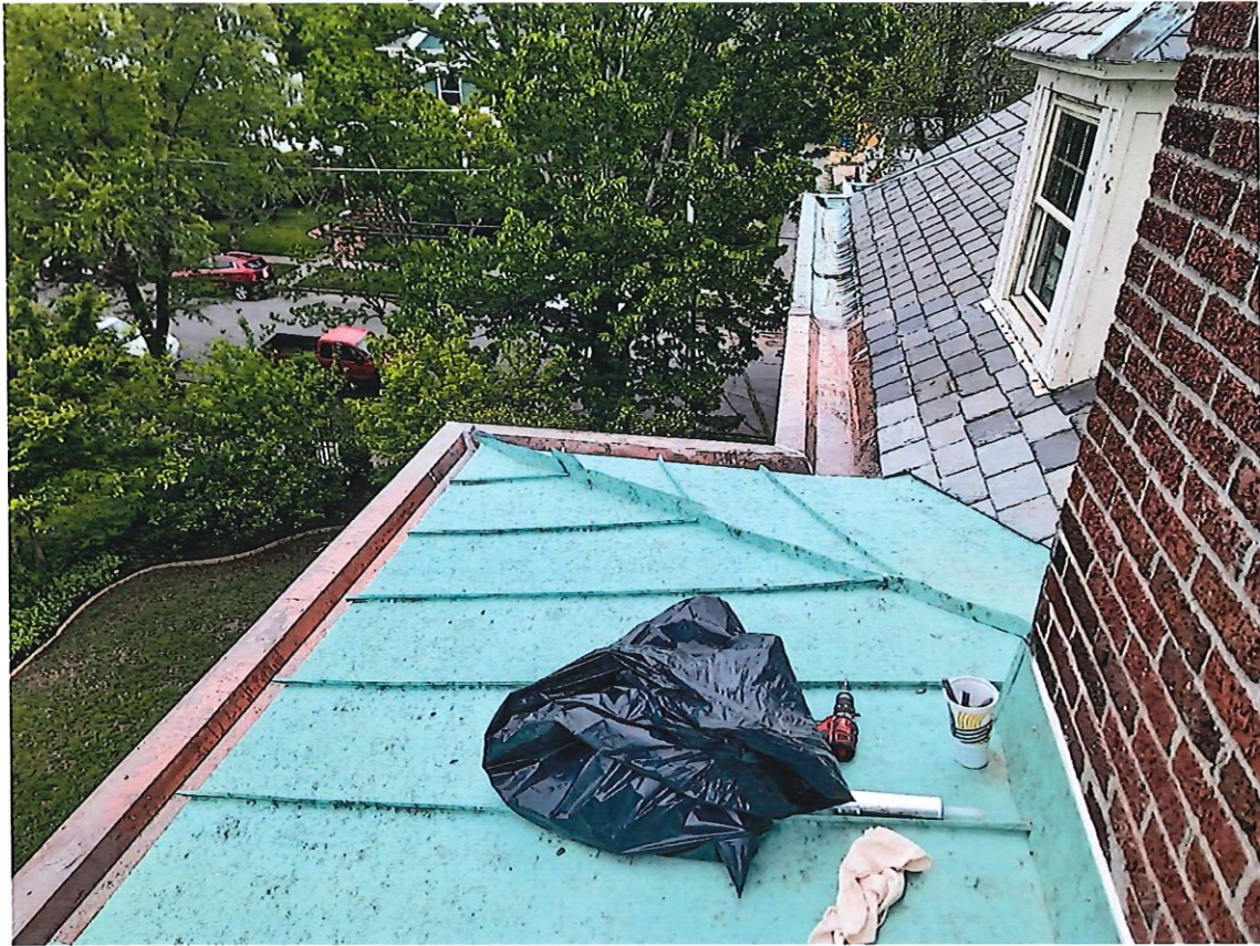
204 Bay Avenue Roof Pictures After Work Completed
