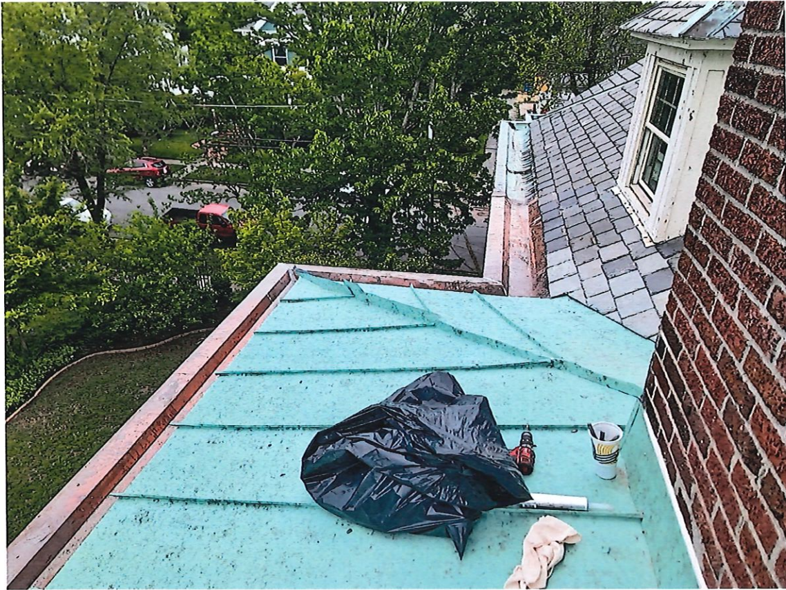
204 Bay Avenue Roof Pictures After Work Completed
