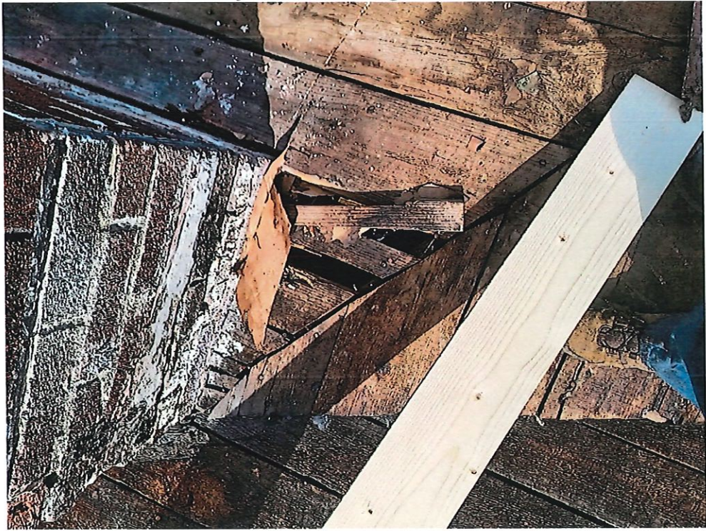
204 Bay Avenue Existing Roof Pictures
