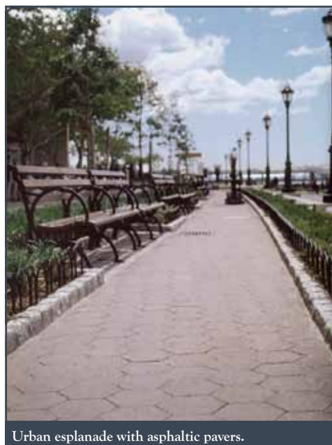
Urban esplanade with asphaltic pavers.
