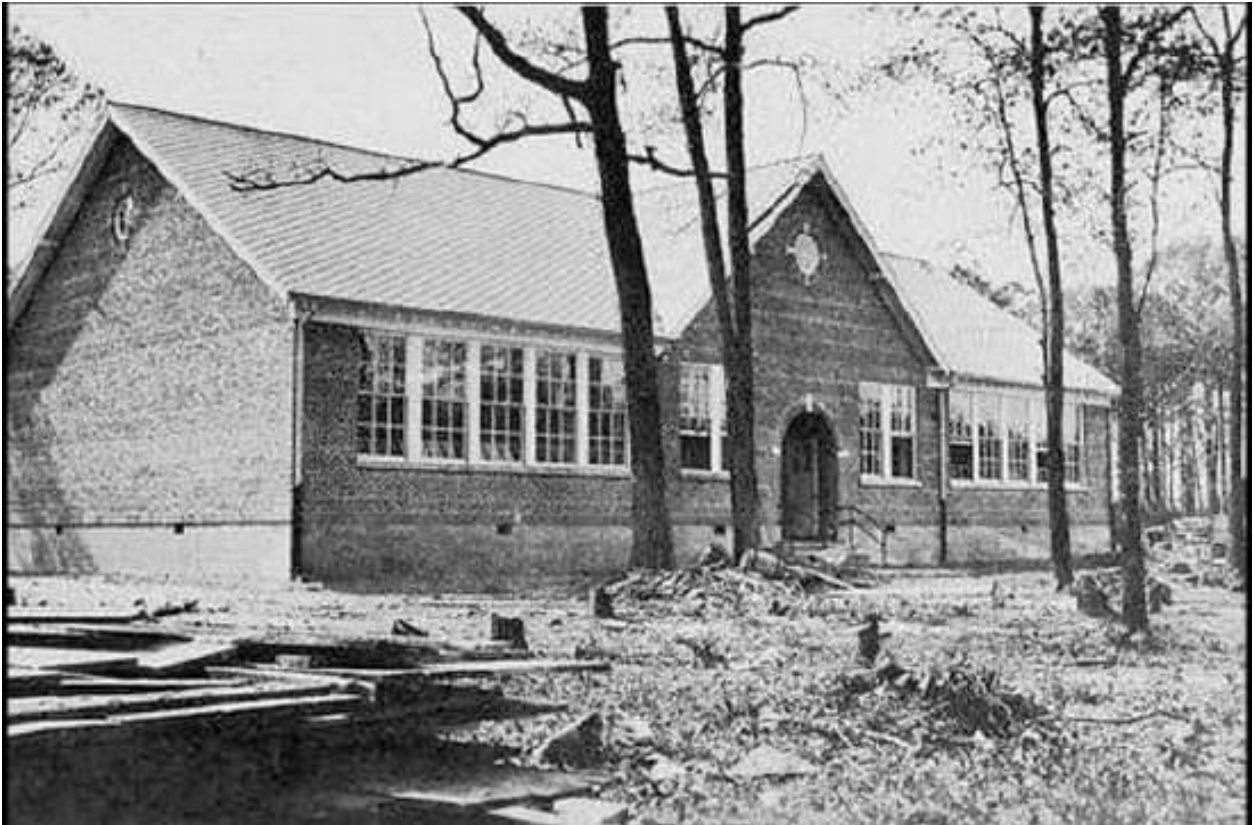
Cape Charles Elementary School – Historic Photo Circa 1929 - View from the Southeast (Photographer Unknown)
