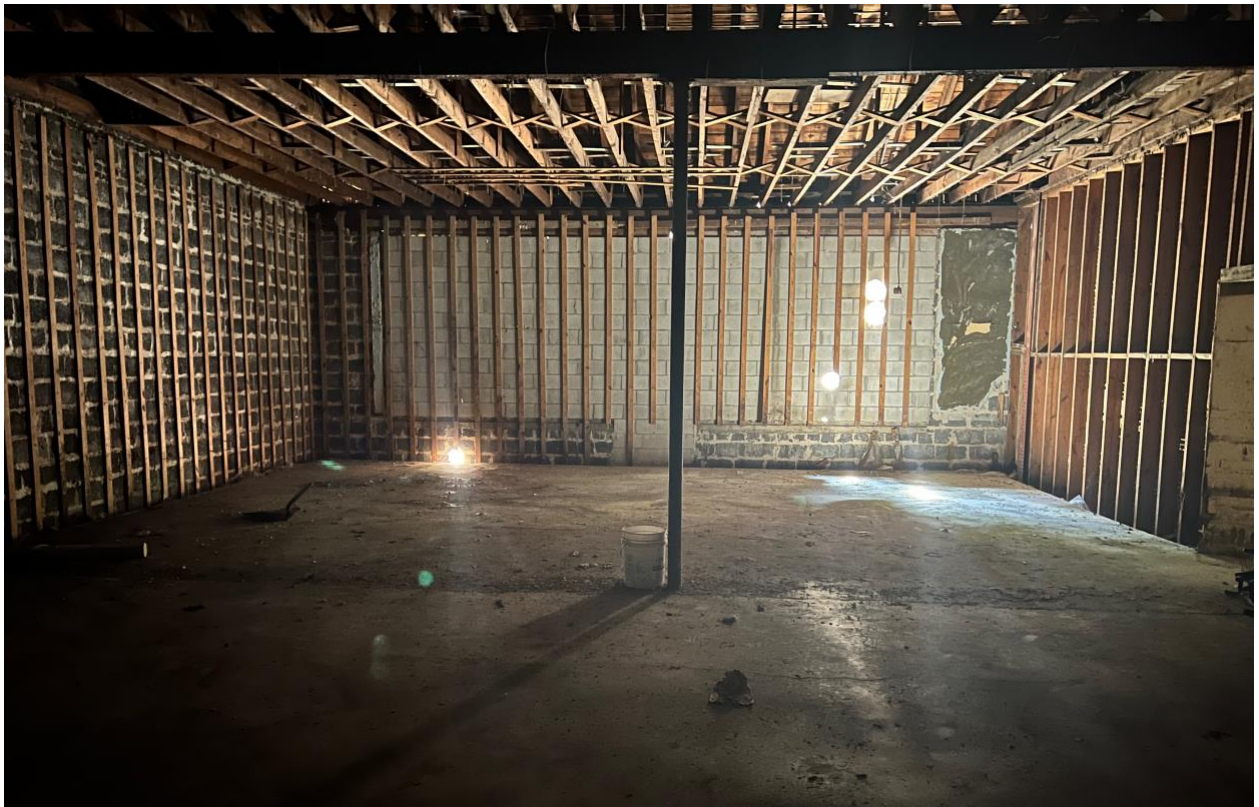
Cape Charles Elementary School – Interior View of Southern Classroom (Courtesy of B. Walker)
