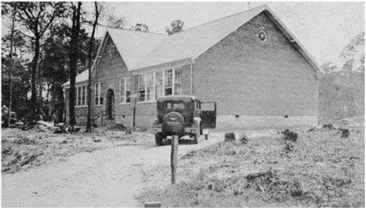
Cape Charles Elementary School – Historic Photo Circa 1929 - View from the Northeast (Photographer Unknown)
