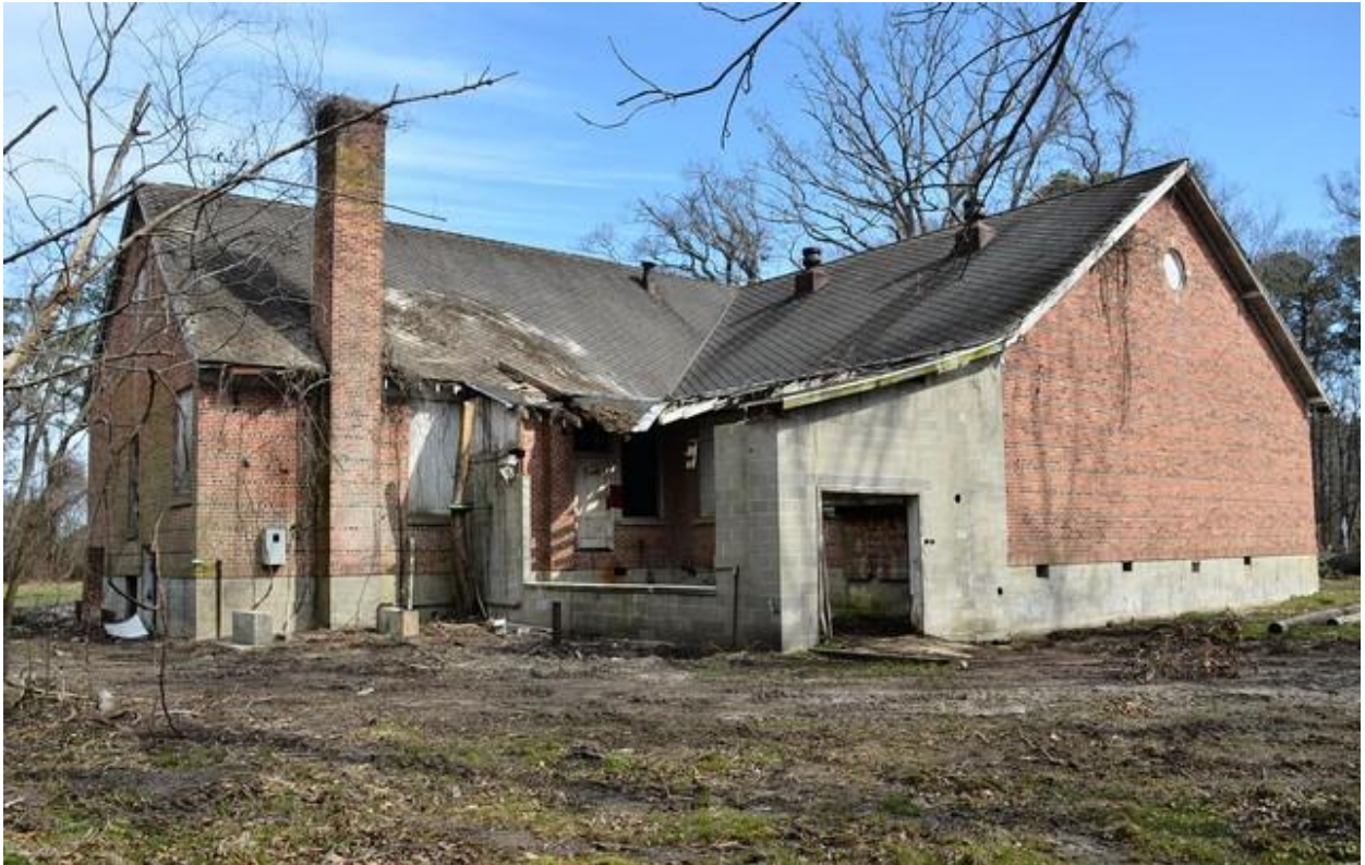
Cape Charles Elementary School – View from the Southwest (Courtesy of The Patina Group)
