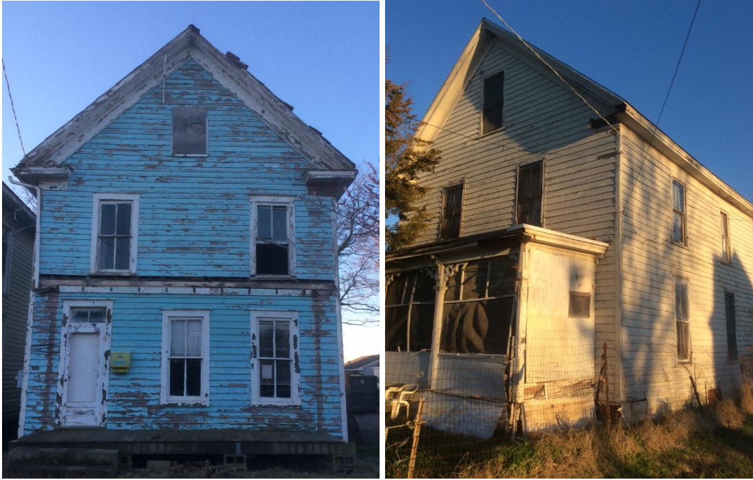
Derelict Houses in Danger of Demolition, (Larry Dire, March 2019)
