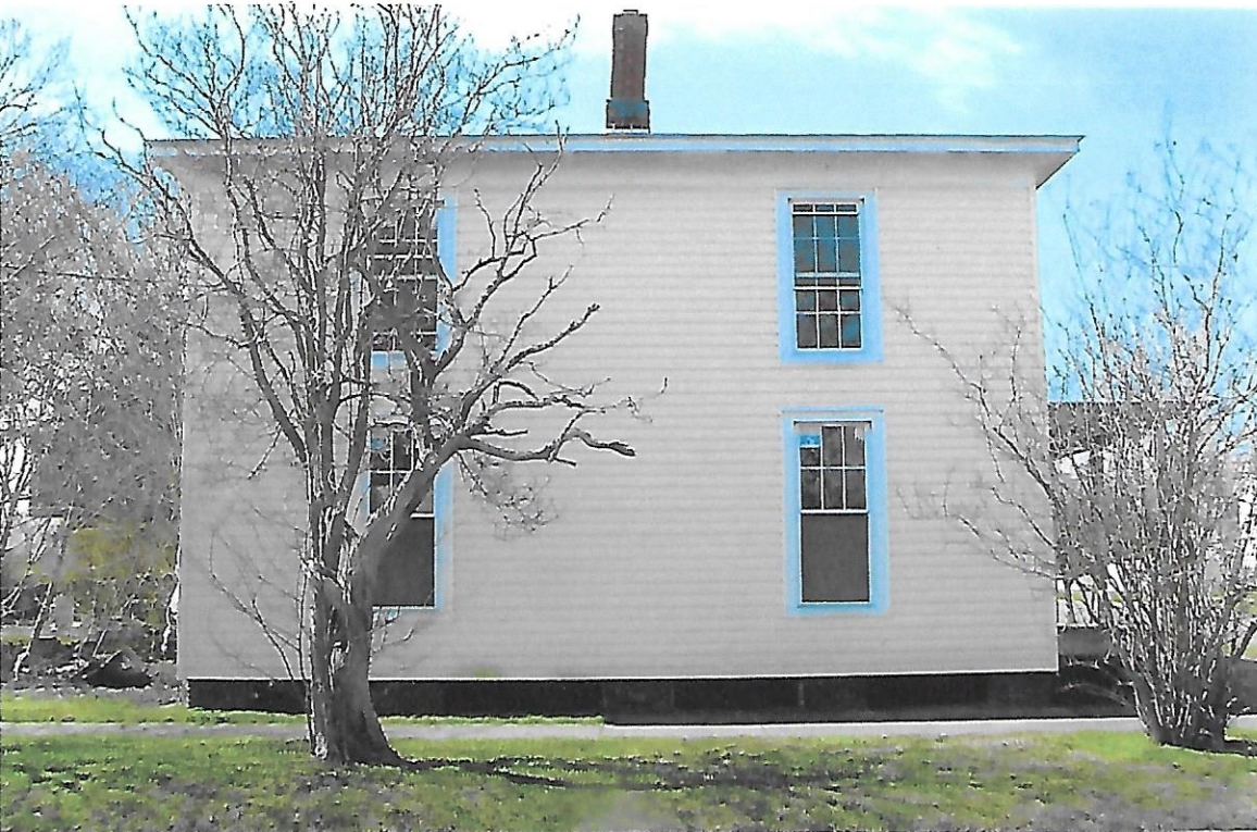
EXISTING LEFT SIDE ( EAST ) FROM PLUM STREET
