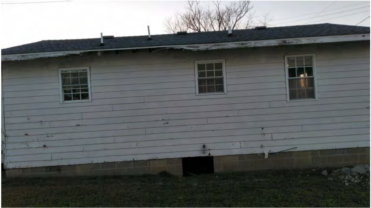
Photos of existing structure:
