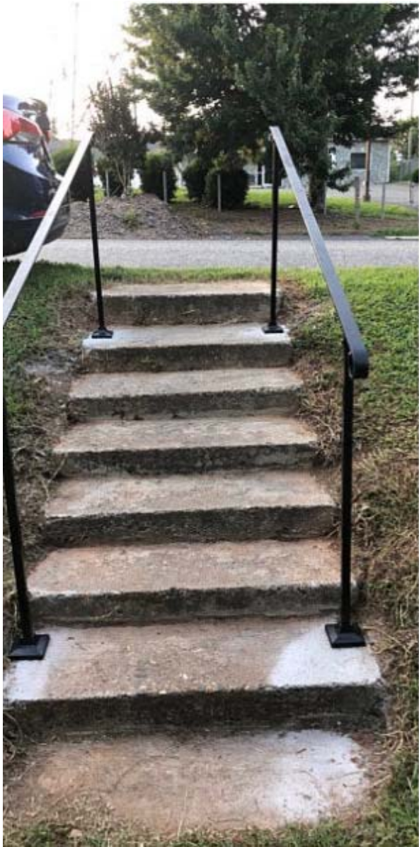
Better image of the longer rails required
