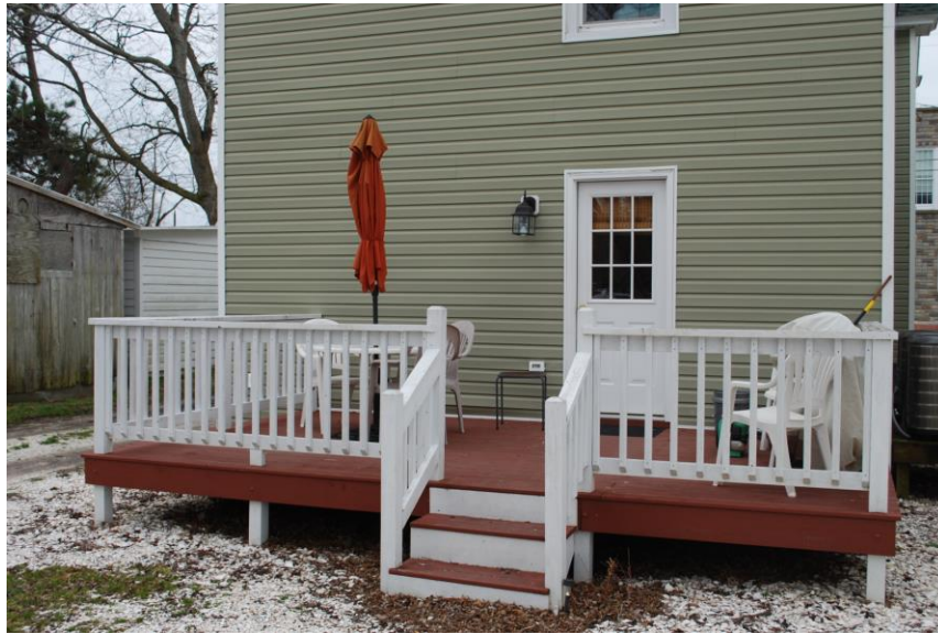
Photos of existing conditions at back yard of 416 Plum Street:
