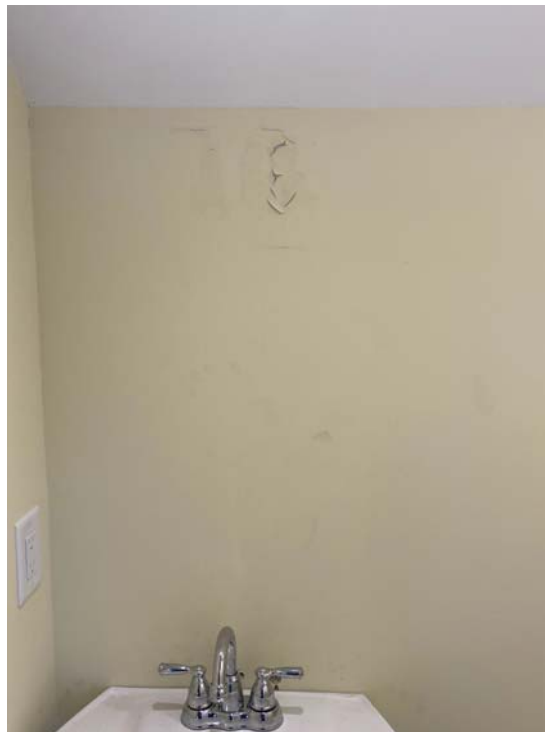
Water damage in 2 nd floor HVAC duct and behind mirror in 3 rd floor bathroom
