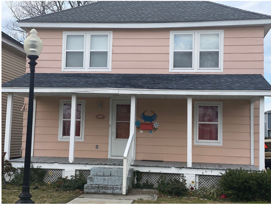
Example of double windows at 609 Peach St
