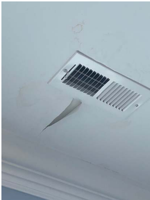
Water damage in 2 nd floor HVAC duct and behind mirror in 3 rd floor bathroom
