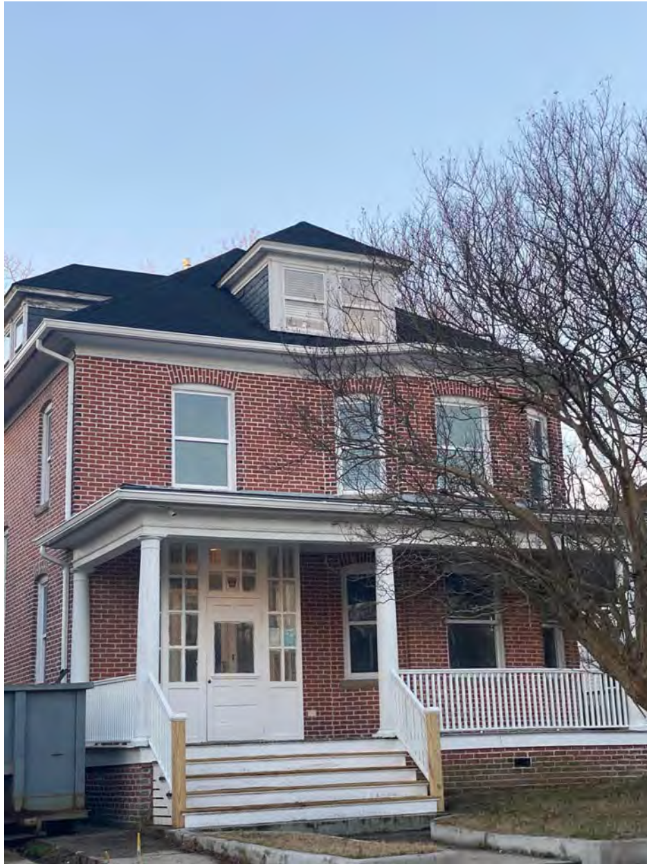
This is our house with the new roof
