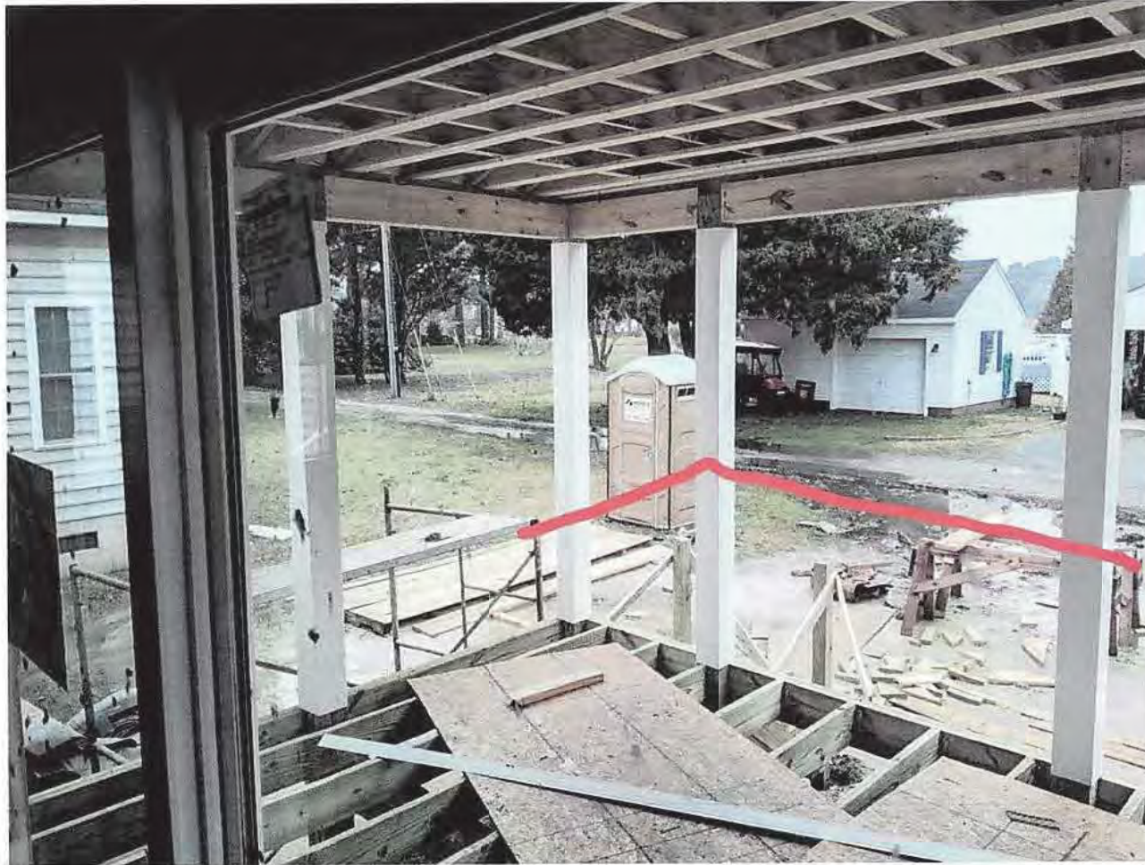
view from inside - Dining room
