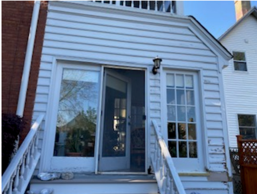
Figure 1 Door and window on south side
