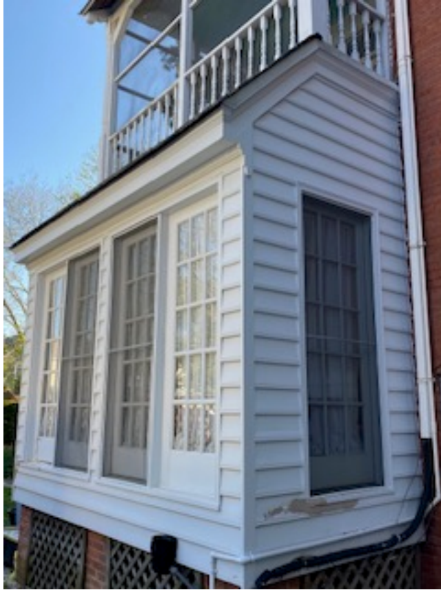
Figure 4 Northeast corner of porch
