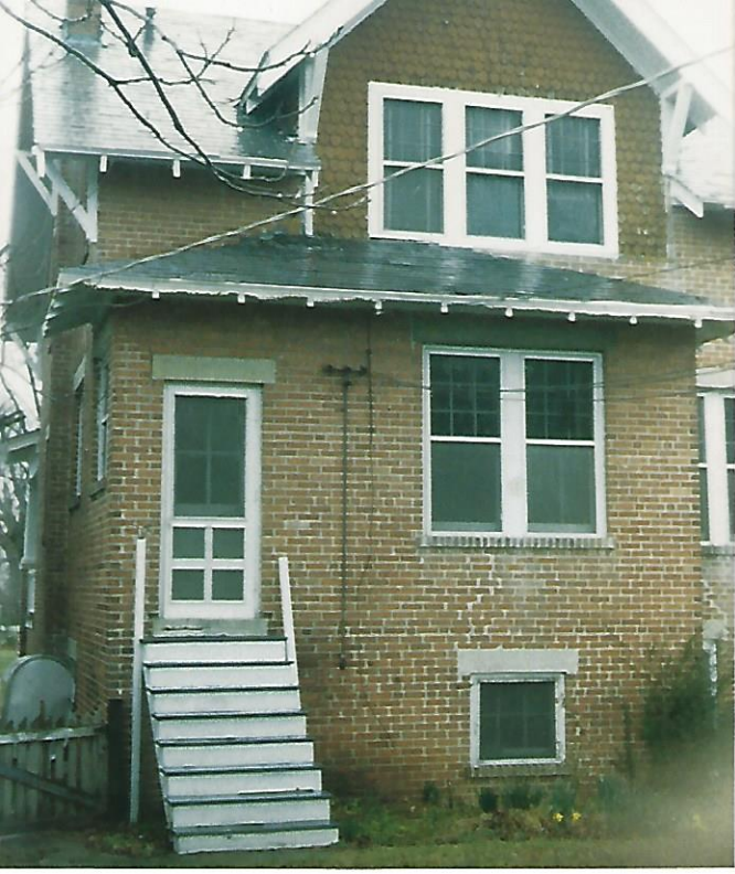
ORIGINAL BEFORE RENOVATIONS
