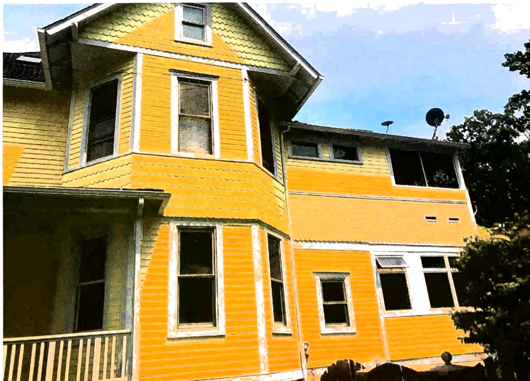
RIGHT SIDE [WEST SIDE] OF HOUSE
