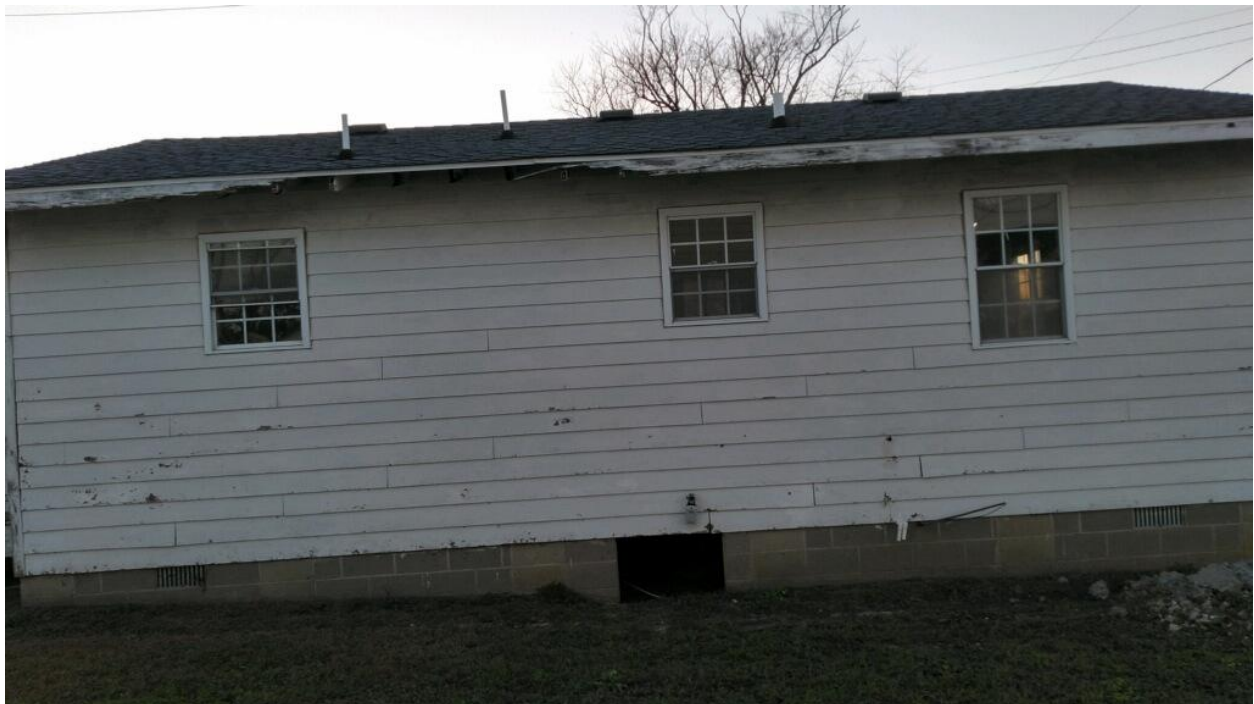
Photos of existing structure:
