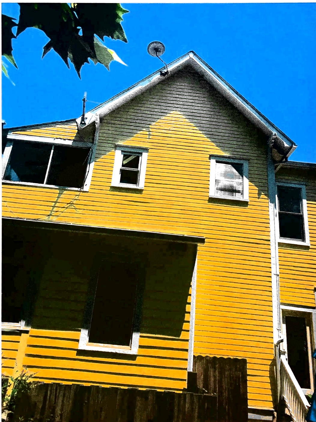
REAR OF HOUSE - SOUTH SIDE
