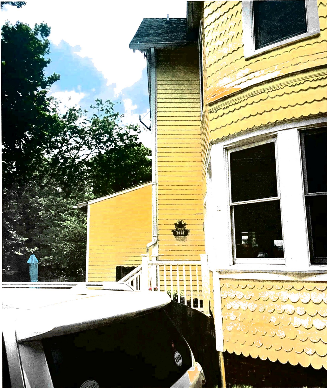
LEFT SIDE [EAST SIDE] OF HOUSE FROM DRIVEWAY
