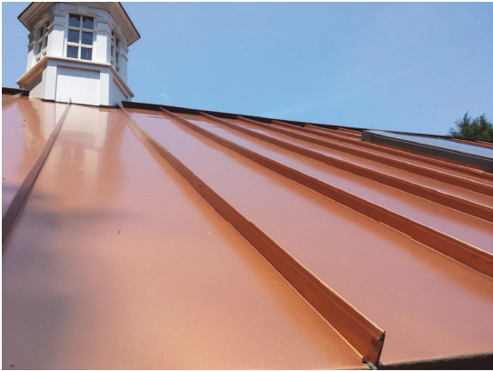
STANDING SEAM ROOF. (FOR DETAIL ONLY)
