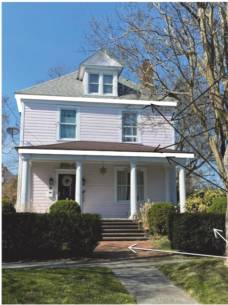
FRONT OF HOUSE (LOOKING NORTH)
