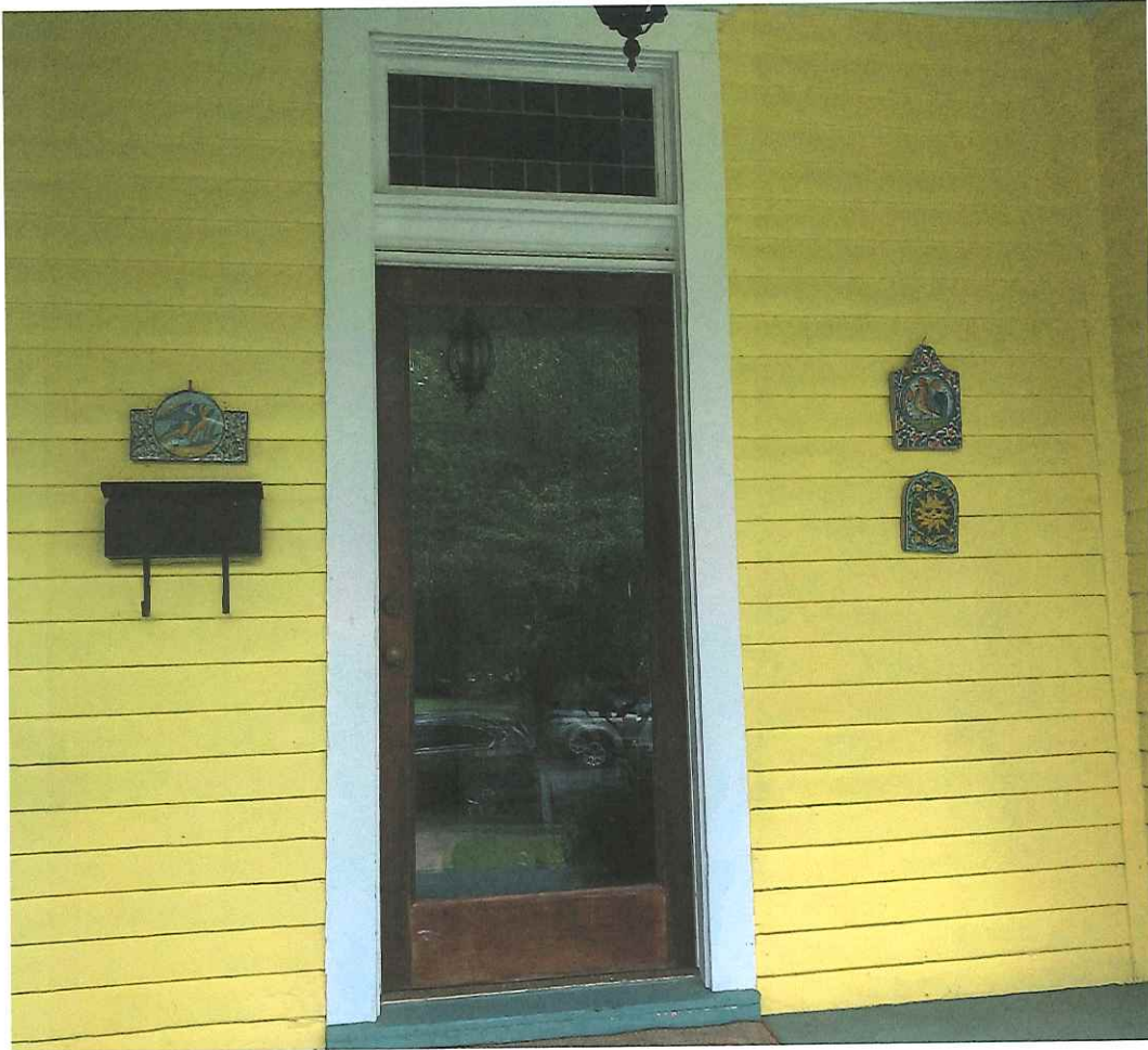
EXISTING FRONT DOOR TO BE REPLACED
