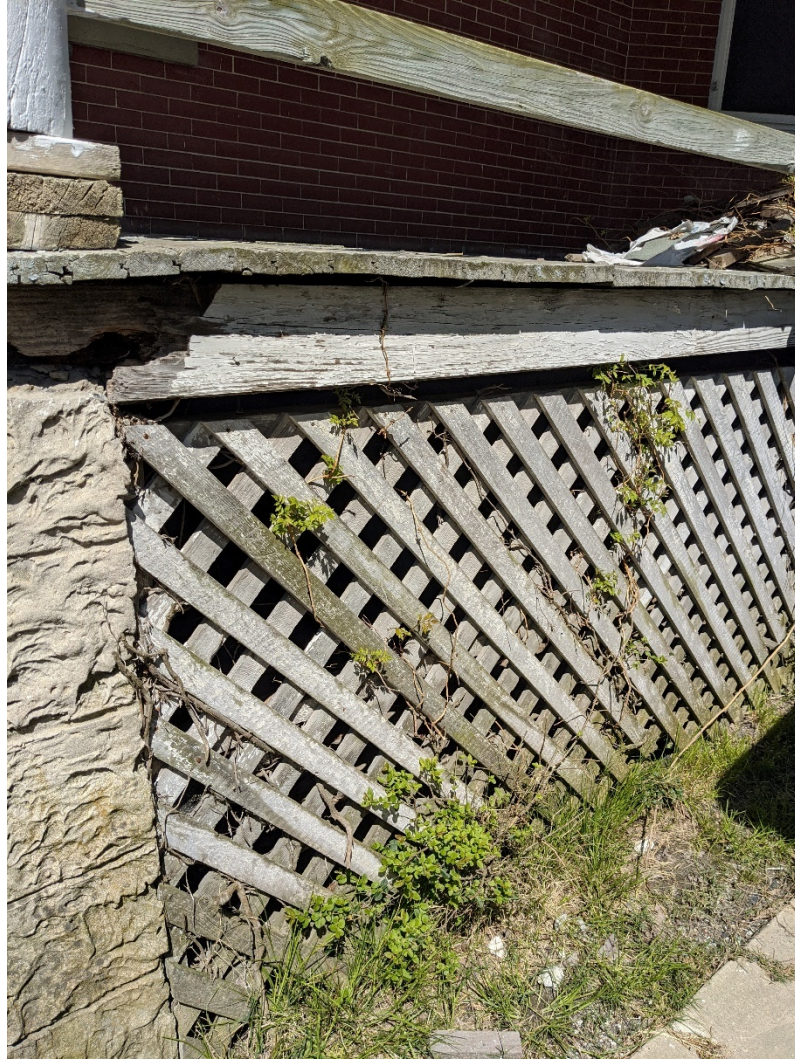
Figure 6-1A: Displaying currently standing and installed lattice.
