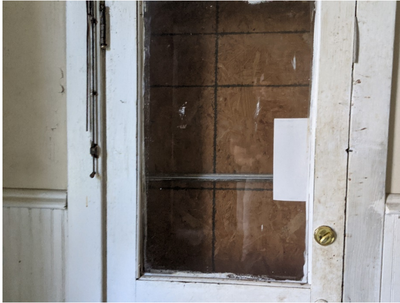
Figure 3-1A: Shows a white-painted wooden door with glass panes already installed within the rear of the home at time of assessment.
