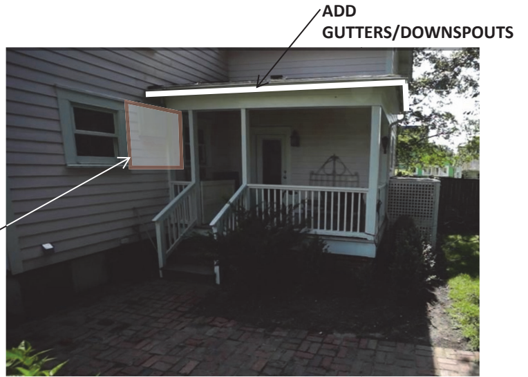
REAR OF HOUSE (LOOKING WEST)
