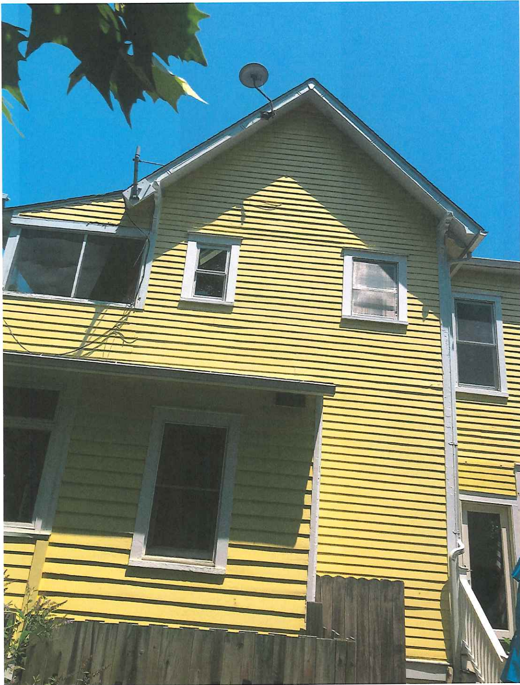
REAR OF HOUSE - SOUTH SIDE
