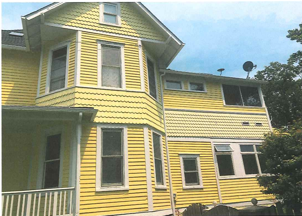
RIGHT SIDE [WEST SIDE] OF HOUSE
