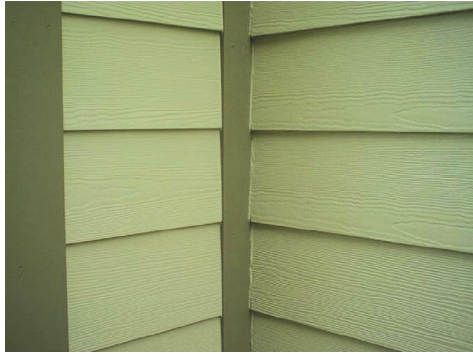
TYP. SIDING VIEW - WOOD GRAIN FINISH, 7" FACE
