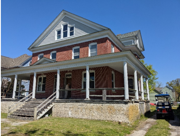
Figure 2-1A: No picture from atop the roof was taken, main picture used as reference for roof.
