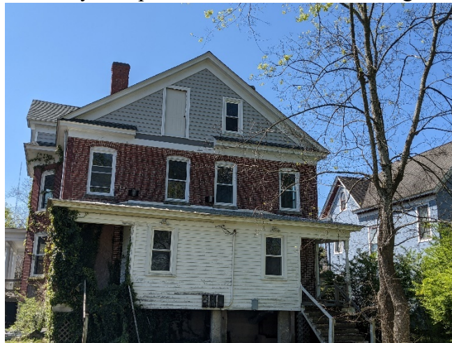
Figure 4-4A: Showing windows that may need minor touchup, along with the door to be replaced with a window that will need trim to harmonize.
