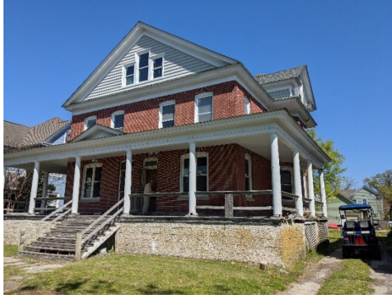
Figure 3-2A: Outside view of the front of the residences to display the exterior windows condition.
