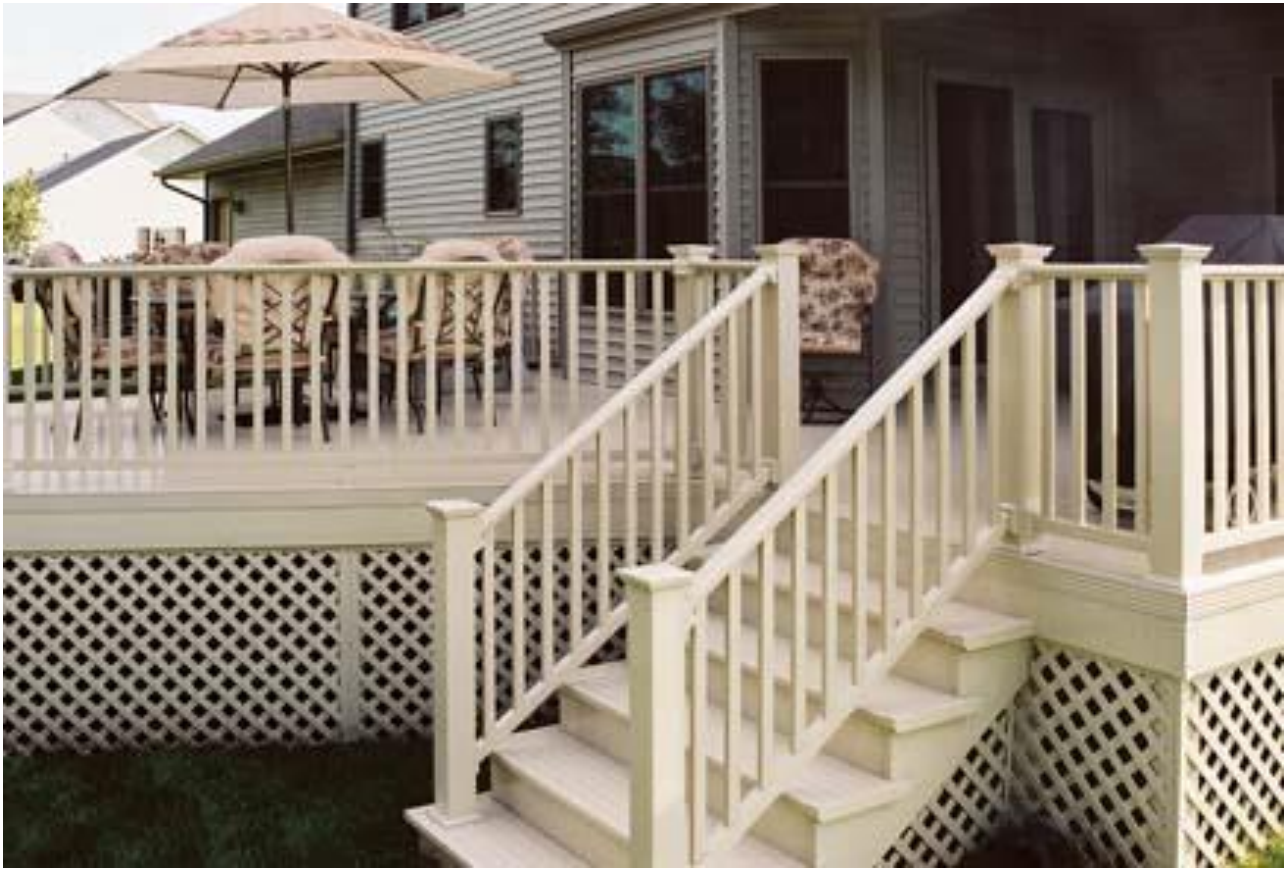
White: Porch stair handrails
