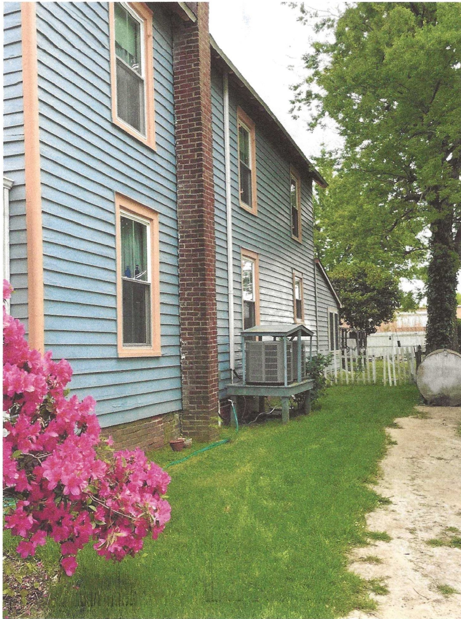
East side of house. New fence would be in same footprint as current fence, 75 feet from front
