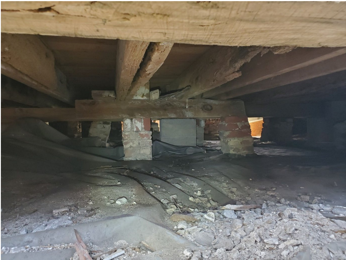
Foundation, joists, beams
