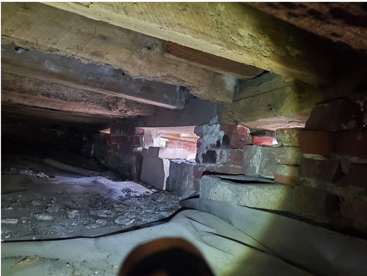
Foundation, joists, beams
