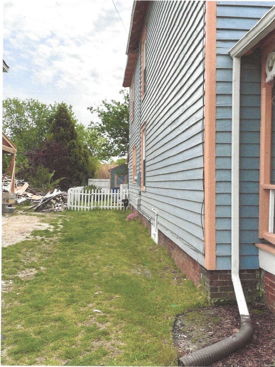
East side of house. New fence would be in same footprint as current fence. Fence would sit 75 feet from front of property line
