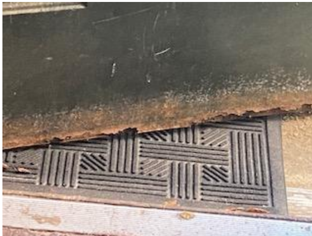
Low threshold for wheelchair
