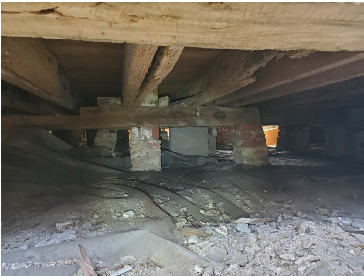
Foundation, joists, beams
