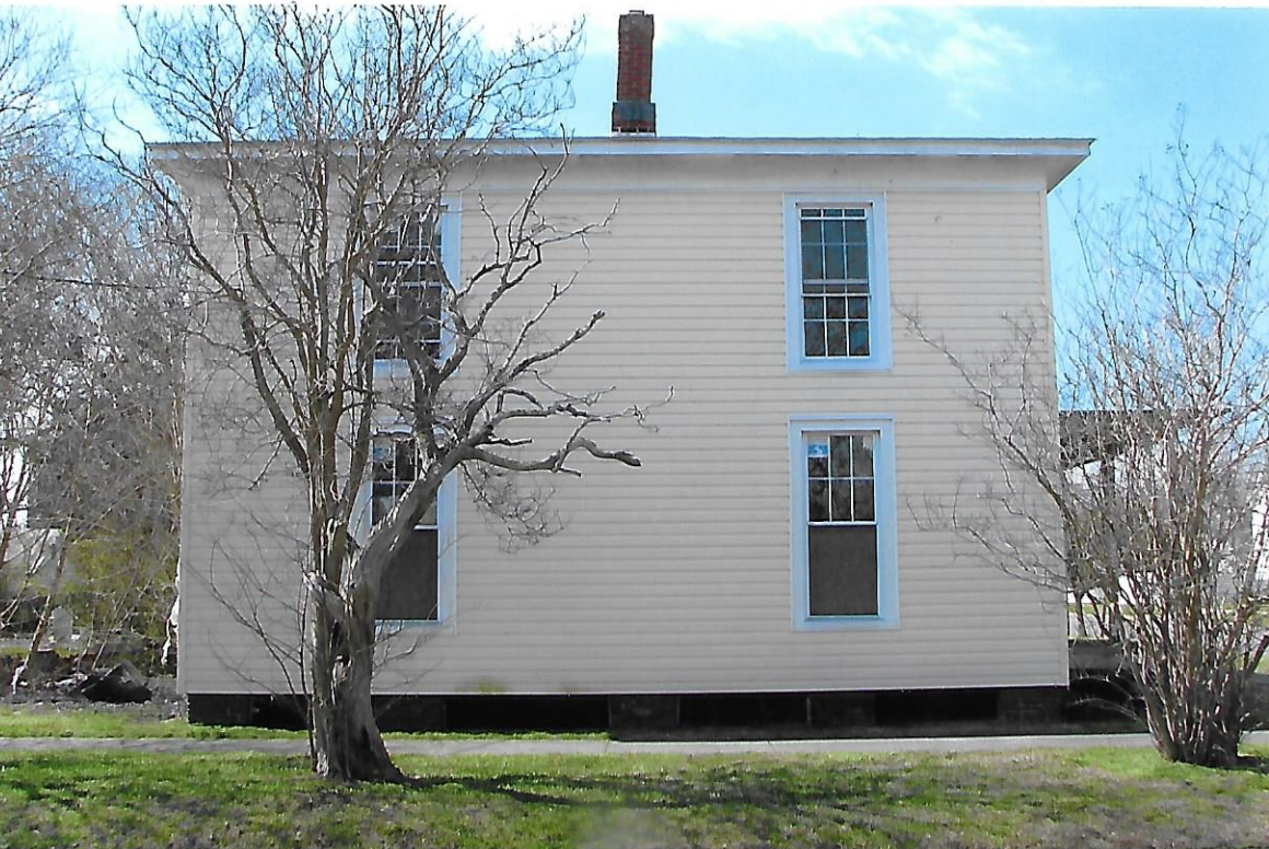
EXISTING LEFT SIDE ( EAST ) FROM PLUM STREET
