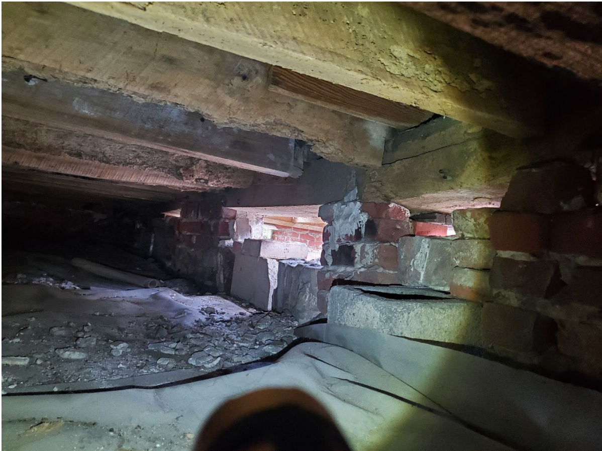
Foundation, joists, beams
