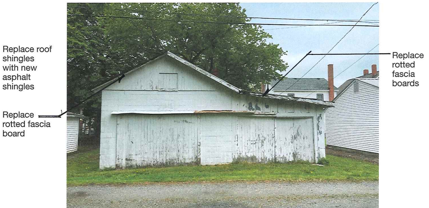
Existing Garage Building from Alley
