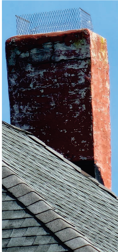
Furnace Rear Chimney
