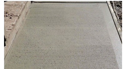
GREY, BROOMED, CONCRETE, WALKWAY
