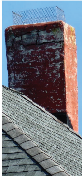
Furnace Rear Chimney
