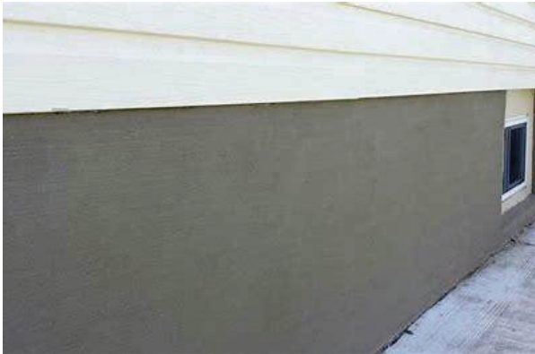
GREY PARGED CMU BLOCK FOUNDATION
