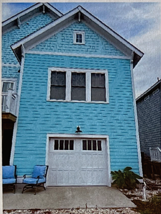
Existing Garage Door (#7)
