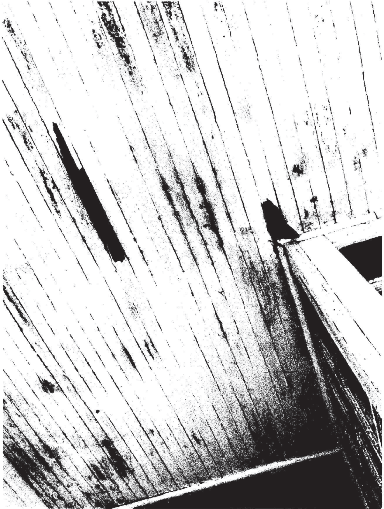
Front Porch Rot
