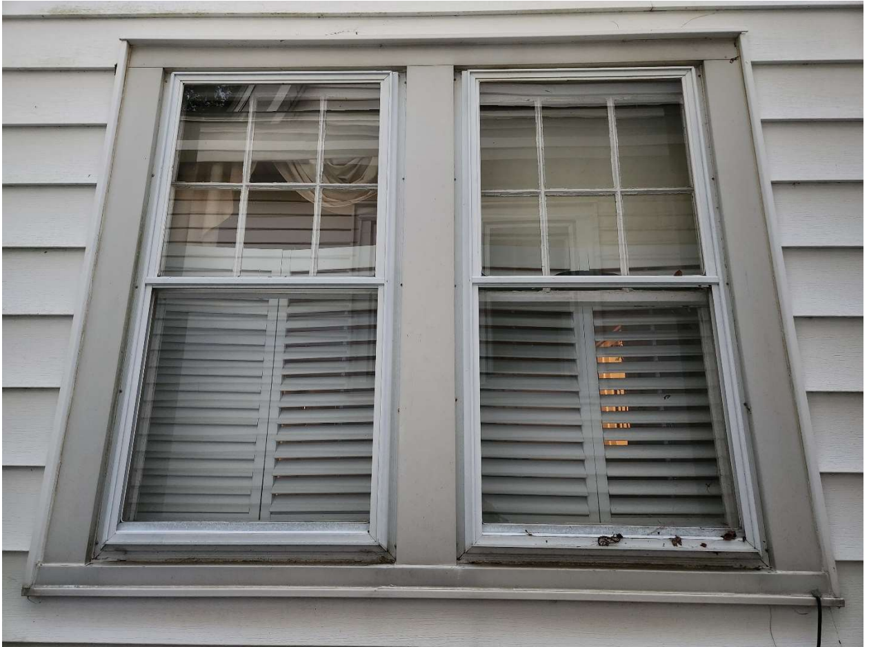
212 Madison – 1 st Floor Existing Windows (Typical)
