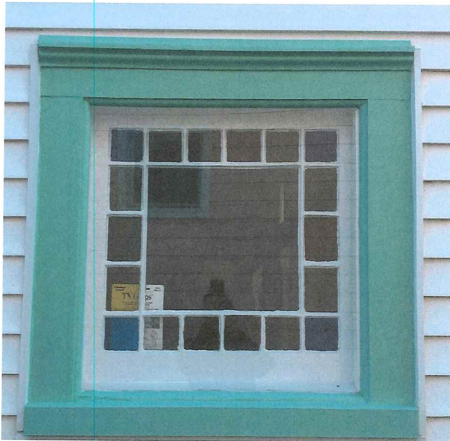
Existing Window Trim Detail To Be Matched with Azek
