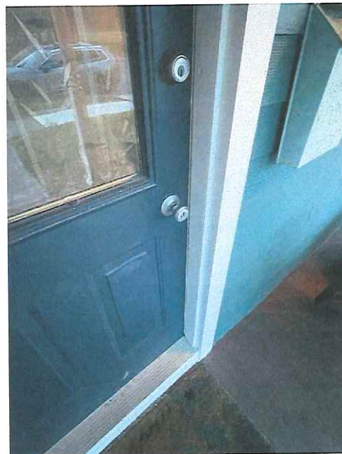
Existing, damaged, modern metal front door.
