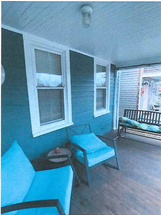
Existing vinyl first floor façade windows. façade.
