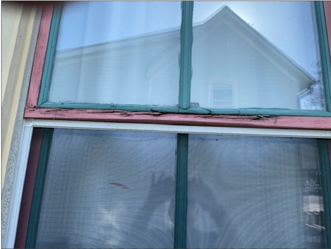
519 Mason Avenue Existing Window Pictures
