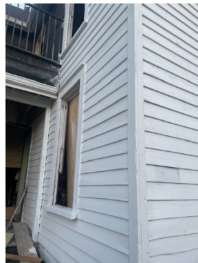
Figure 6 Left side of the house after demo and prime
