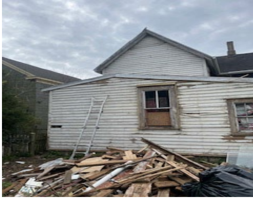
Figure 1 Back of the house after Demo
