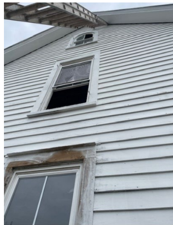
Figure 5 Left side of home after demo and prime
