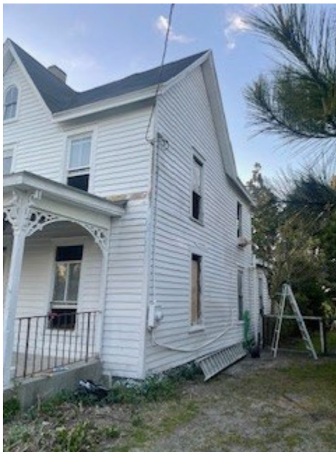
Figure 2 front and right side of the home after demo and prime
