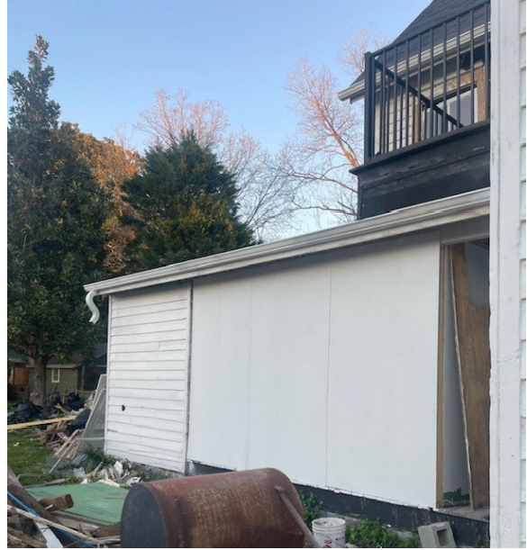
Figure 4 Left side of home after demo and prime
