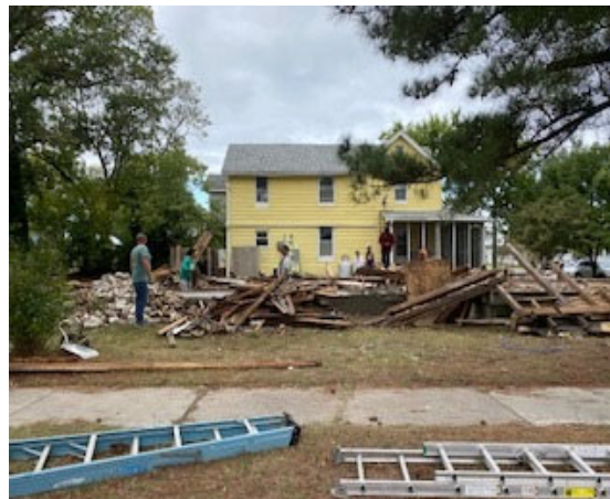
Lot Immediately after Demolition – 10/13/2021
