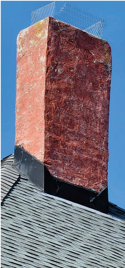
Fireplace Front Chimney
