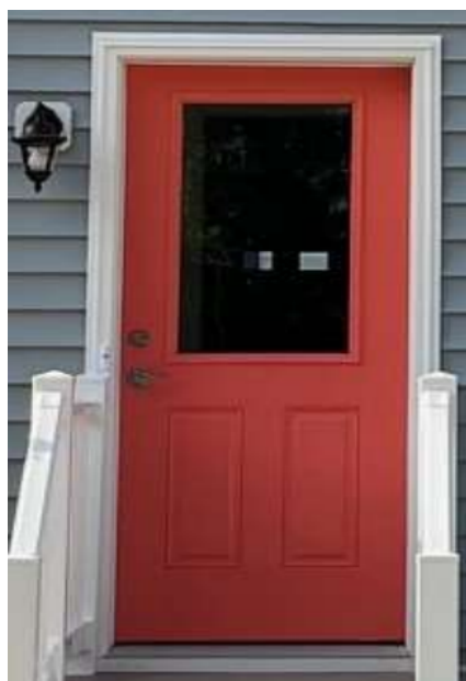
Rear Door (off of Mud Room)
