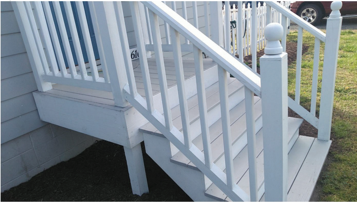
Porch Balustrades and Columns – Pressure Treated Wood (Example Below) Square 2 X 2 Pickets, 2 X 4 Rails, 4 X 4 Columns
