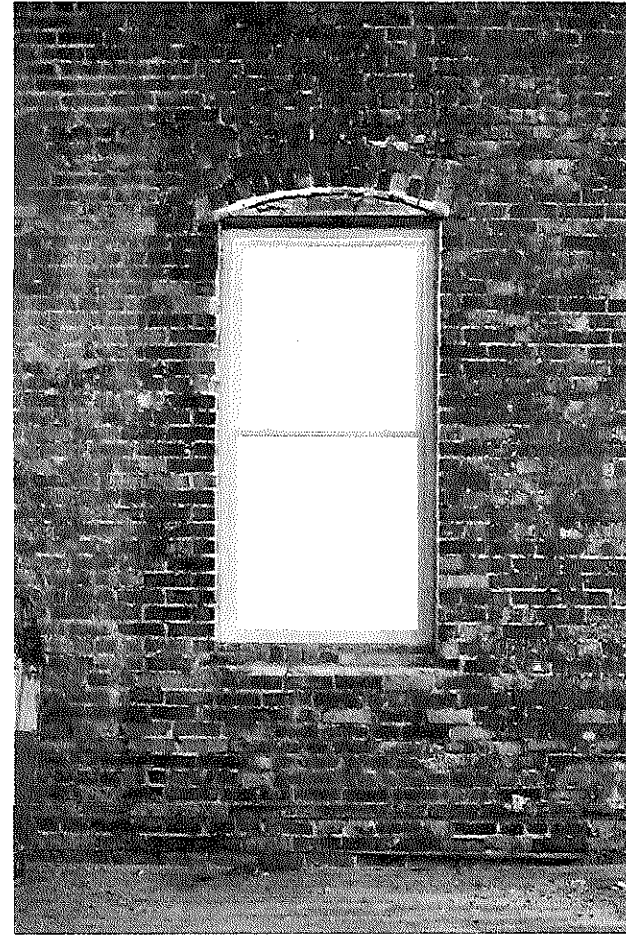
Interior photos showing exterior brick to be re-pointed, cleaned, and exposed within the units. Depending on condition, brick to be painted or sealed with clear sealer. This photo also shows the existing rack arches above some window openings, which are to be retained and exposed.
