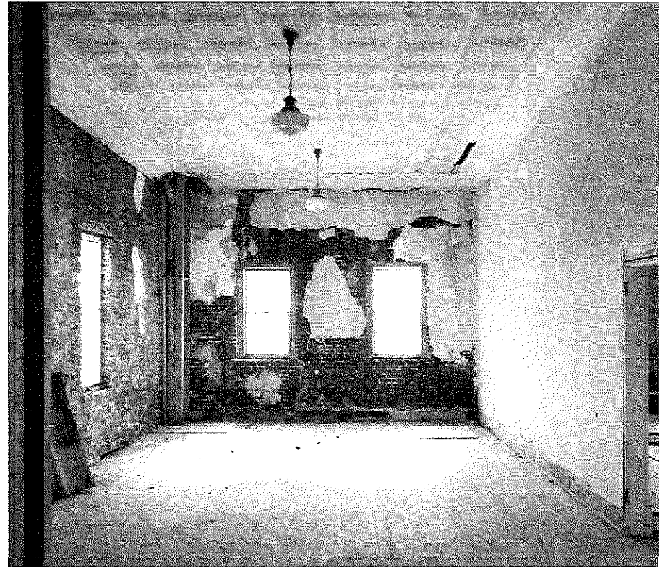
Current photo of existing interior condition. The existing tin ceilings (in good condition) are to be salvaged and re-used in the retail spaces.
