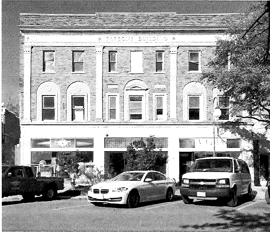
Current photo of existing front facade
