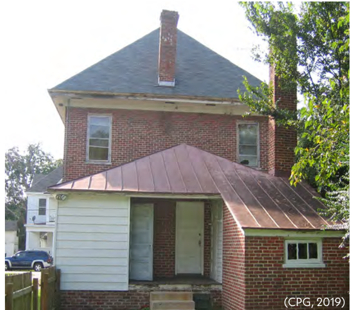
Figure 5.11 - The primary chimney (left) should be retained as long as it is structurally sound. The secondary chimney (right) may be proposed for removal as it is secondary and not visible from the public right-of-way.
