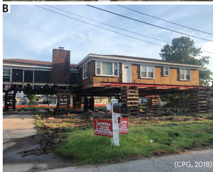
Figures 8.11 A & B - Elevating a historic home significantly alters its appearance and historic materials (A). It is also an extremely costly and delicate procedure and should be a last-resort measure for historic buildings (B).
