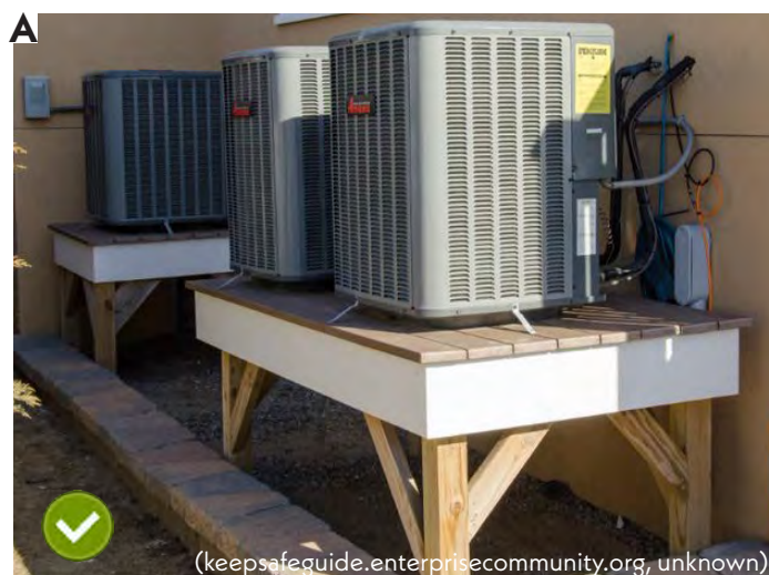
Figure 8.9 - A diagram of raising mechanical systems from FEMA's "Reducing Flood Risk to Residential Buildings that Cannot be Elevated" publication.
