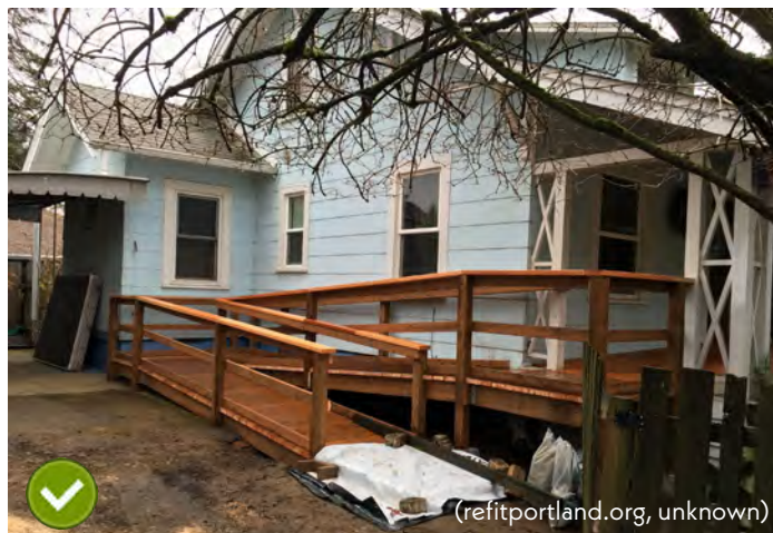
Figure 9.7 - This ADA ramp is sympathetic to the building's historical design. It is simple in design and material and placed along a secondary elevation with access to front porch from the side. If it is eventually removed, the balustrade can easily be replicated and reinserted.
