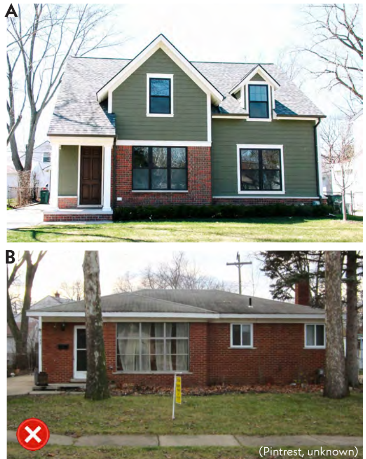
Figures 5.43 A & B - The drastic alteration (A) to this one-story ranch house into a two-story residence overpowers the form and scale of the original primary building (B). It also borrows many historic features, giving it a false sense of history.
