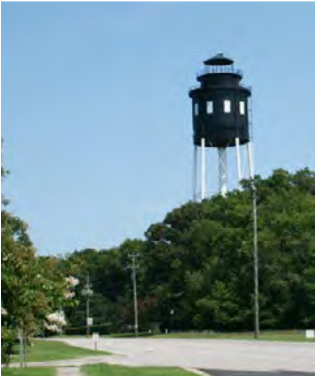
Cape Charles water tower.
