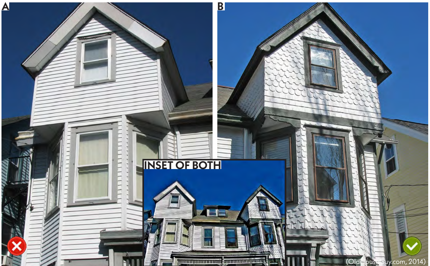
Figures 9.13 A & B - The rowhouse on the right retains its historic wood shingles, decorative trim, and exposed rafter tails. The rowhouse on the left has been completely covered in vinyl siding. All ornamentation has been removed and the character defining features lost to the detriment of the individual resource and character of the overall Historic District. Alternative materials should be applied thoughtfully and only when necessary.
