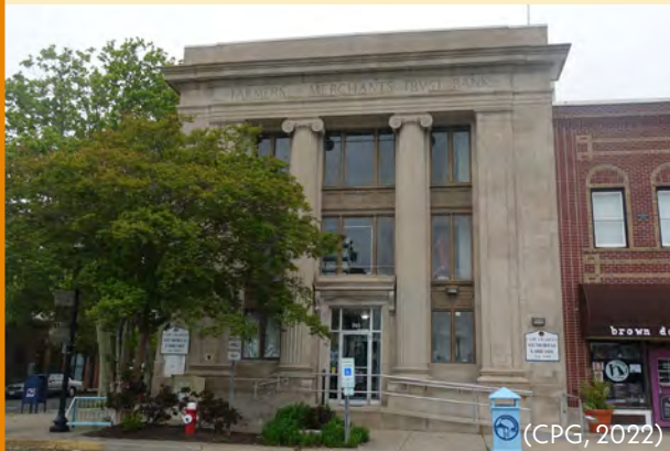
201 Mason Ave (Institutional Building)
