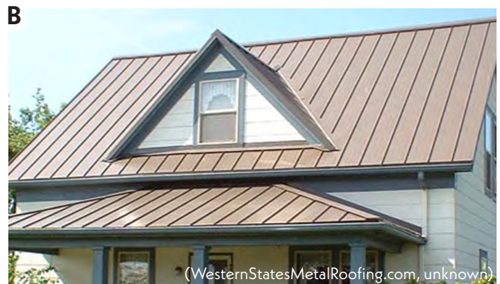
Figures 4.2 A & B - The top photograph is an example of a pressed metal roof, while the bottom illustrates a metal standing seam roof.
