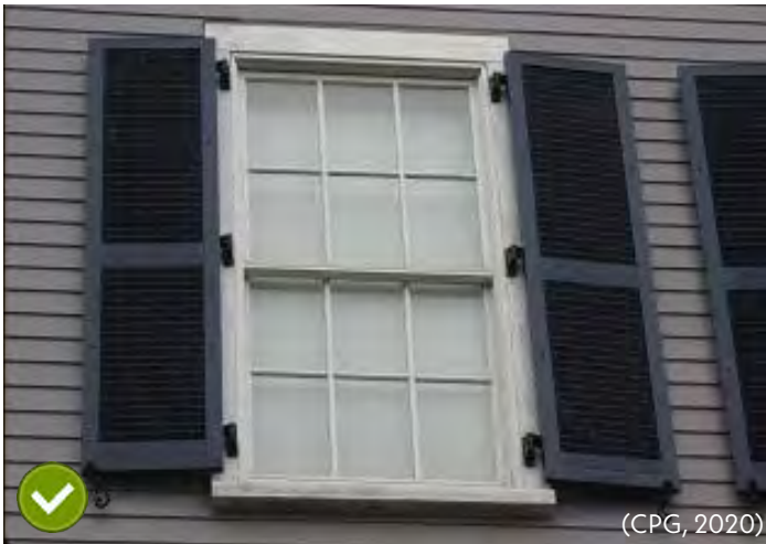
Figure 5.23 - The shutters above are clearly operable with hinges and holdbacks. They also protrude slightly away from the wall, showing depth. These are appropriate shutters for a historic building.
