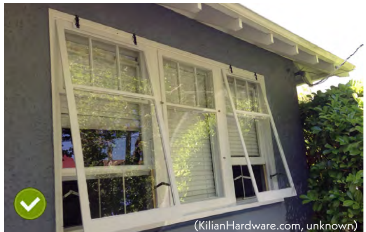
Figure 5.25 - These storm windows have a frame and meeting rail that matches the window, as well as paint color that matches the wood frame.
