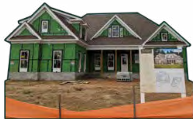
Home under construction in Bay Creek.
