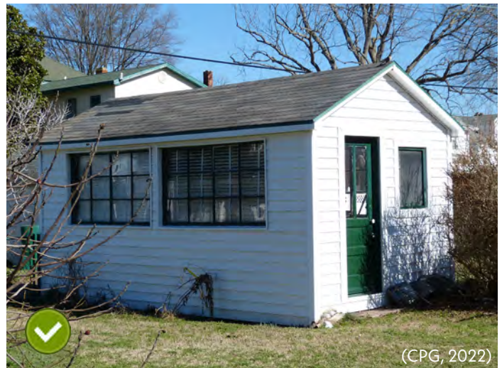
Figure 6.2 - An example of a well-maintained noncontributing accessory structure associated with a contributing primary building in Cape Charles.
