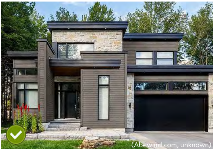
Figure 7.4 - This noncontributing house has been clad in Hardi-plank siding. It is differentiated from historic materials found in the Cape Charles Historic District and would be appropriate on a noncontributing building.
