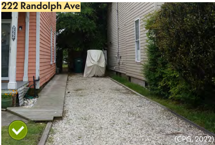
Figure 9.1 - Compacted oyster shells or pebbles are appropriate materials for new driveways. They help mitigate water issues with their porous surface, promoting better drainage.
