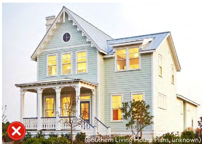
Figure 5.40 - This new building utilizes too many details that replicate historic details such as the gingerbread trim on the eaves, the fishscale shingles on the wall, and the porch trim.
