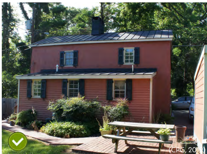
Figure 5.34 - This addition at the rear of the building is appropriately subordinate to the historic building. The wood siding also differentiates it from the painted historic material used on the original building.
