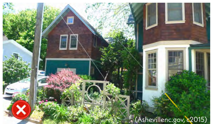
Figure 6.1 - This garage has been converted to an ADU. The addition matches the historic home closely, creating a false historic narrative. It is also substantially larger now and along a public right-of-way, impacting the integrity of the site and primary resource.
