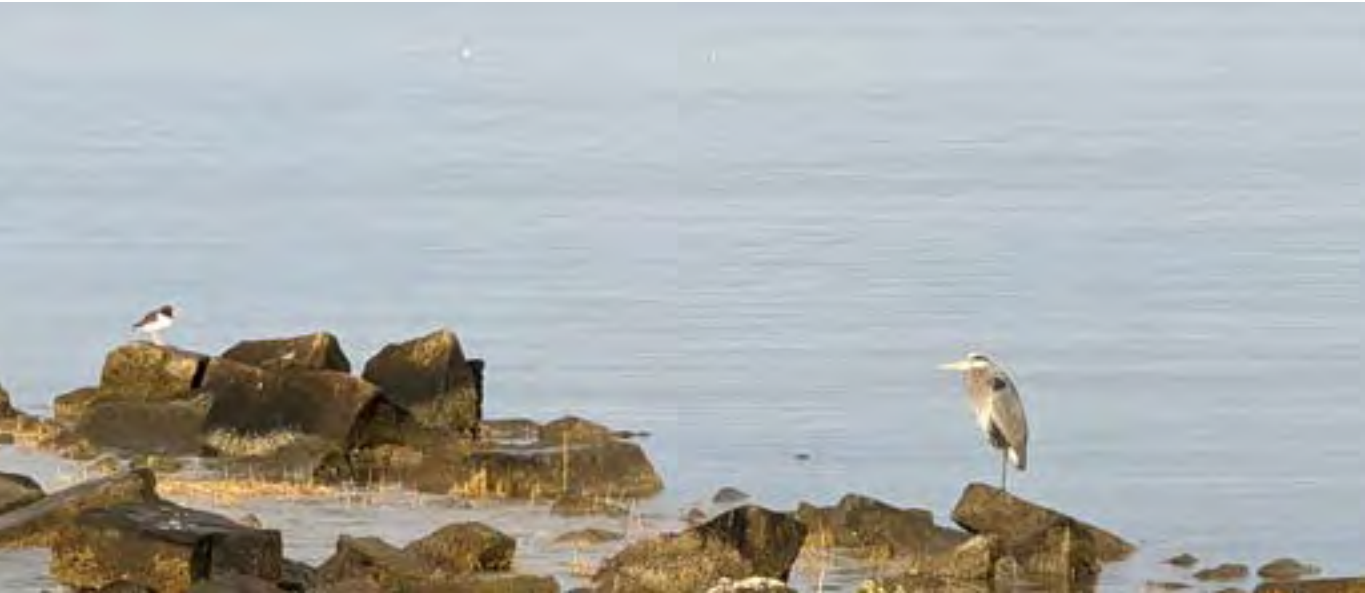
Birds perched at the eroding jetty.
