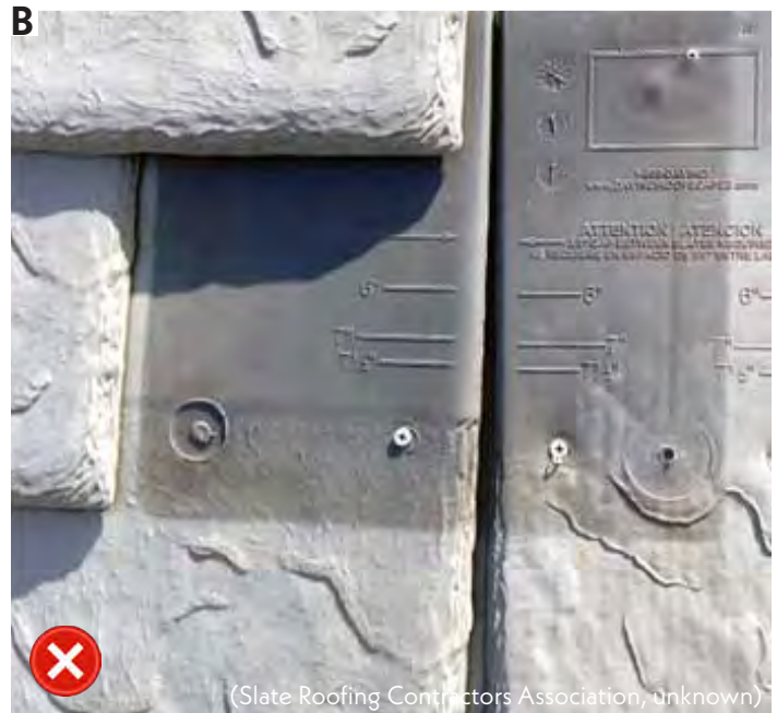
Figures 5.2 A & B - Synthetic slate roofing is not an appropriate replacement material, as it has a tendency to warp (A), pucker, and bleach (B).
