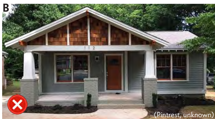
Figures 5.39 A & B - The addition of a Craftsman style front porch (defined by the use of wood shingles, deep eaves, exposed rafter tails, and thick wood columns) to this Minimal Traditional style home is inappropriate.
