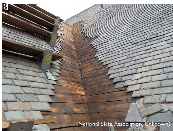
Figures 2.2 A & B - Replacing a few broken or missing pieces of material, like slate tile (top), will save time and money by avoiding large costly projects such as a total-roof replacement (bottom), as well as foregoing the need to obtain a COA. Creating a regular maintenance inspection schedule will help detect these types of repair needs before it's too late.
