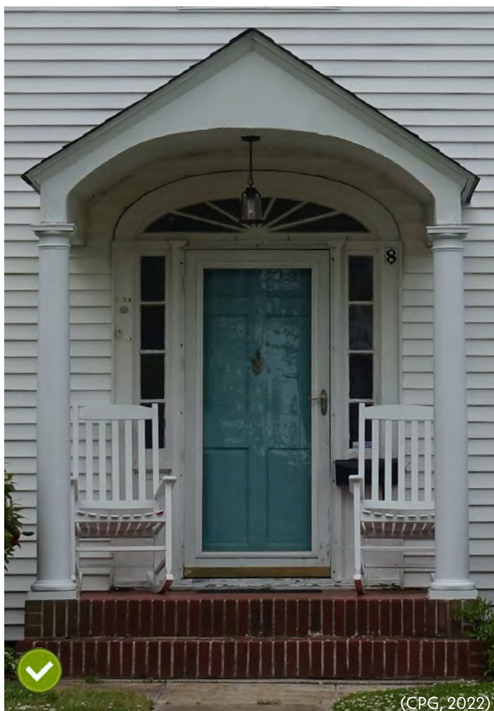
Figure 5.27 - This is an appropriate metal storm door that has a finish matching the trim and minimizes obstruction of the door design.
