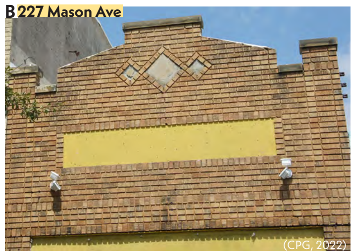
Figures 5.6 A & B - The multiple brick designs on the residential and commercial facades above are character-defining features. They should be retained and remain uncovered.
