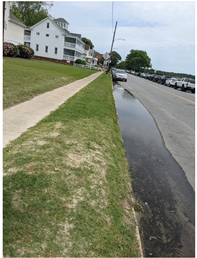
Storm water along Bay Ave. curb.
