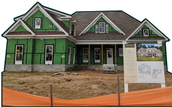
Home under construction in Bay Creek.
