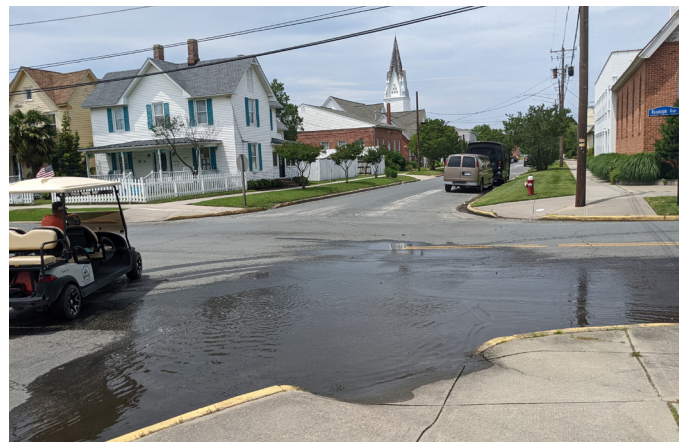
A golf cart drives past the pooled stormwater.
