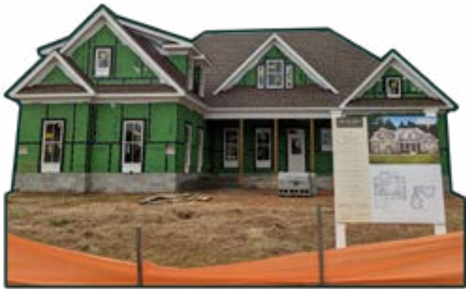
Home under construction in Bay Creek.
