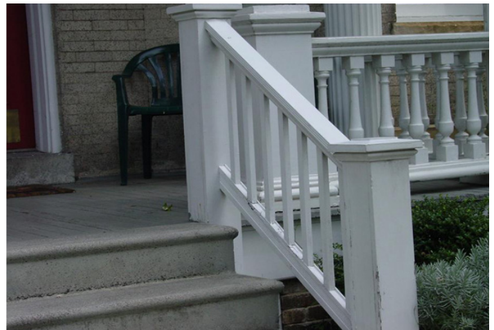
Figure 5.19 - An example of a Richmond rail used on the step railing with the historic balustrade in the background.
