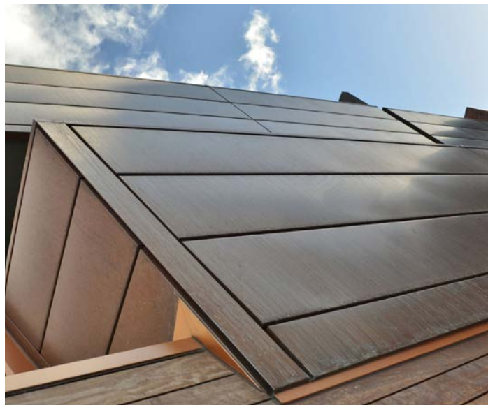
Figure 5.35 - Metal roofing materials now have more design options to give a contemporary look to a noncontributing modern building.
