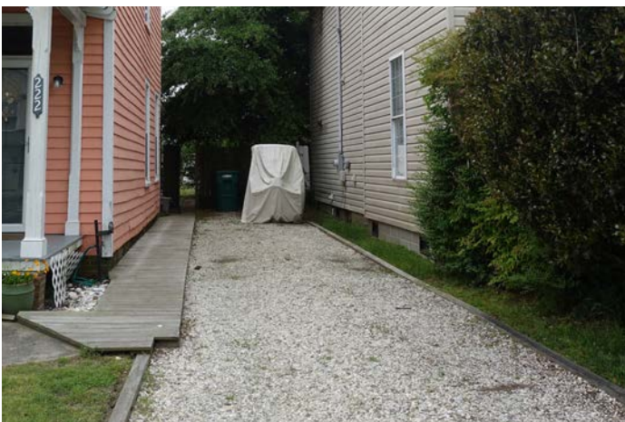
Figure 8.1 - Compacted oyster shells or pebbles are appropriate materials for new driveways. They help mitigate water issues with their porous surface, promoting better drainage.
