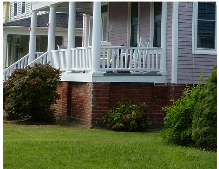
Figure 5.10 - An example of a solid infill to provide additional structural stability. It is recessed between the piers to mark the historic voids.
