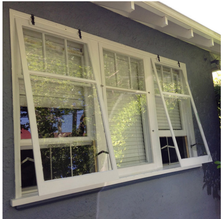
Figure 5.25 - These storm windows have a frame and meeting rail that matches the window, as well as paint color that matches the wood frame.
