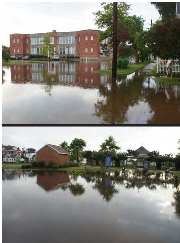
Figure 10.4 - Flooding like the 2017 storm (photographed by the Cape Charles Mirror) could become more common as storms strengthen and sea level rise becomes a persistent issue.
