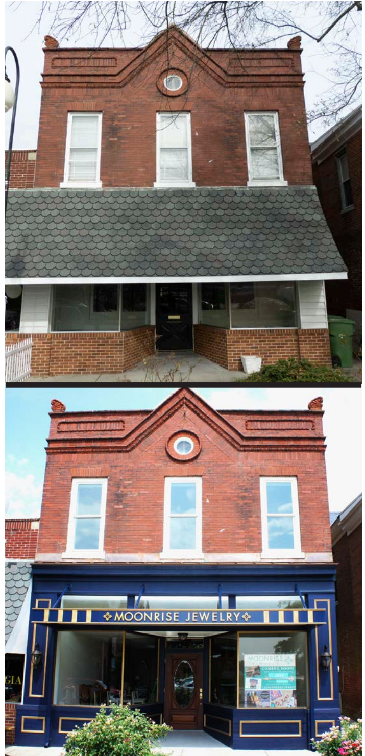
Figure 5.29 - In a recent renovation, the modern shed roof, vinyl siding, and brick veneer knee-wall were removed and a more appropriate storefront was reinstated with transom windows and wood paneled knee-wall and surround. A thin metal awning was added to help manage light infiltration.
