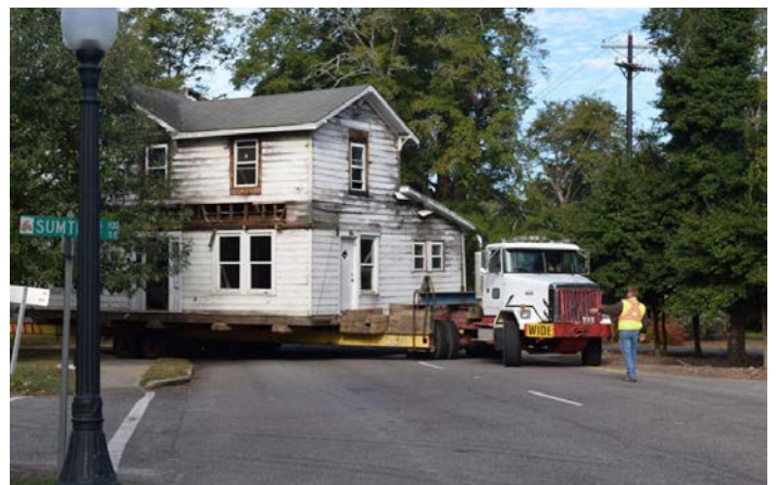
Figure 7.3 - It is a large undertaking to relocate a historic building, and if approved, should be done so with great consideration and planning.
