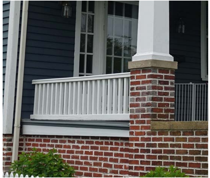
Figure 5.17 - The porch in the above photograph has a gentle slope going away from the building to help keep water infiltration from occurring.
