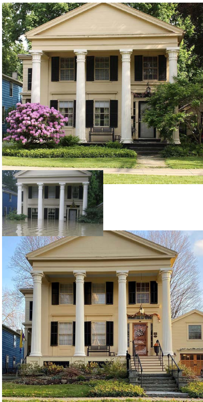
Figure 10.13 - A before (top), during flood (inset), and after elevation (bottom). Notice how the historic building is retained with minimal impact to its appearance. The land has been built up slightly around the property to reduce the height of the lift elevations. Flood vents are strategically placed between the columns, and the new stair is simple in design.
