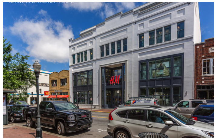
Figure 5.47 - The new commercial infill dwarfs its neighbors and features false-historic design.
