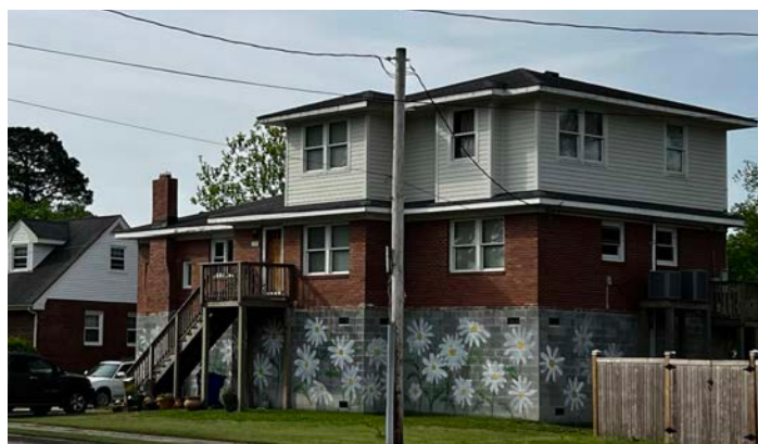
Figure 10.12 - Concrete block is exposed and a new modern stair/deck is disproportionate to the rest of the building. This is a dramatic and visually intrusive solution.
