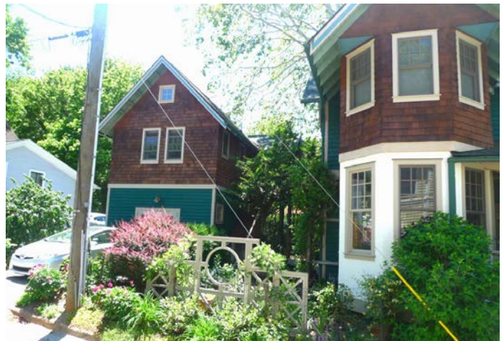
Figure 6.1 - This garage has been converted to an ADU. The addition matches the historic home closely, creating a false historic narrative. It is also substantially larger now and along a public right of way, impacting the integrity of the site and primary resource.
