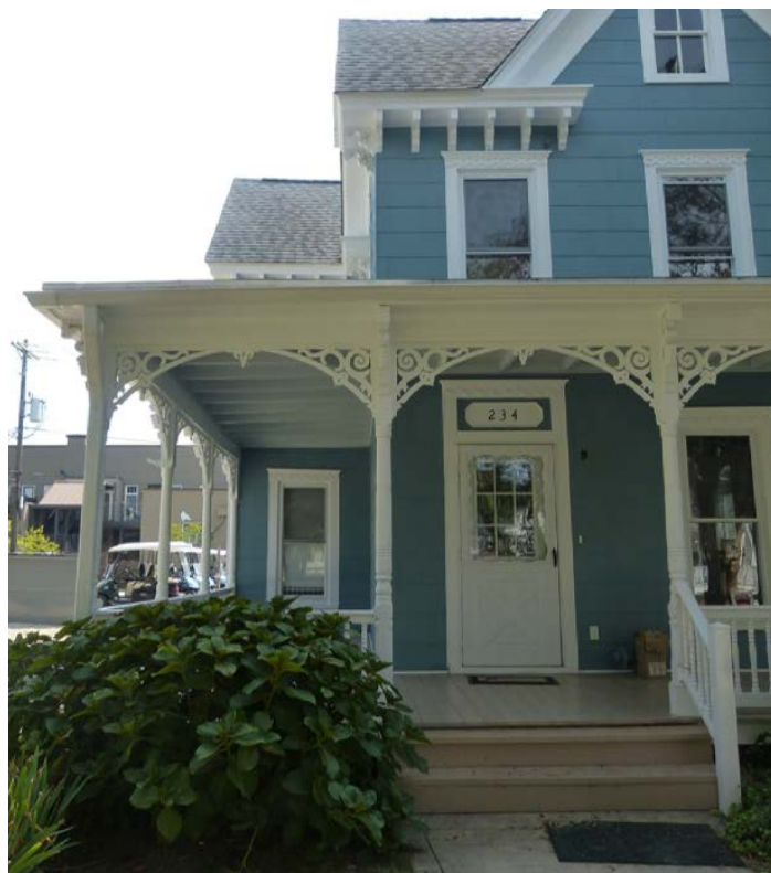
Figure 5.14 - Porches are an important features on many of the Cape Charles residential resources. Their historic design and details should be retained and celebrated.
