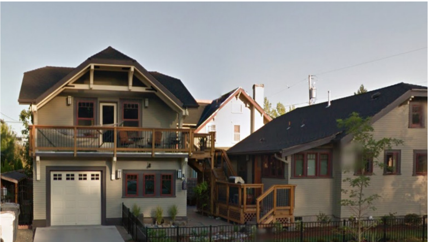
Figure 6.4 - This new accessory structure is placed in the rear yard on a corner lot. It is significantly taller than the primary structure and almost as large. This would be an inappropriate accessory structure in the Historic District Overlay.
