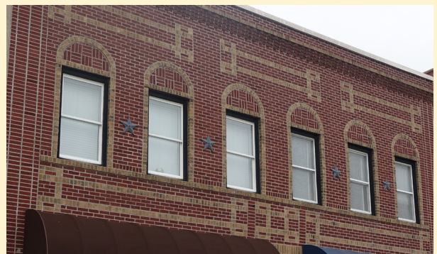
Figure 3.9 - The intricate brick patterning on this commercial facade was performed by highly skilled craftspeople and should be retained as a character defining feature.
