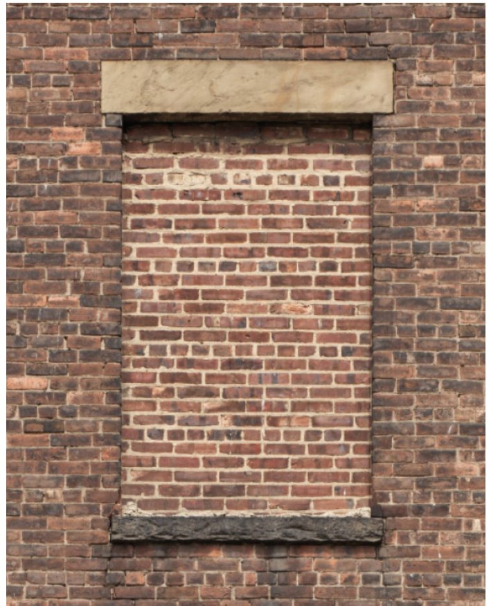
Figure 5.33 - An example of a masonry exterior window infill where the modern brick infill is recessed and the lintel and sill are still present to delineate the historic opening.
