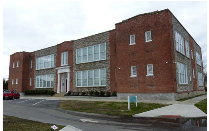
Figure 3.10 - Although currently used as a residential apartment complex, 423 Plum Street is an Institutional building type as it was originally designed as a public school.
