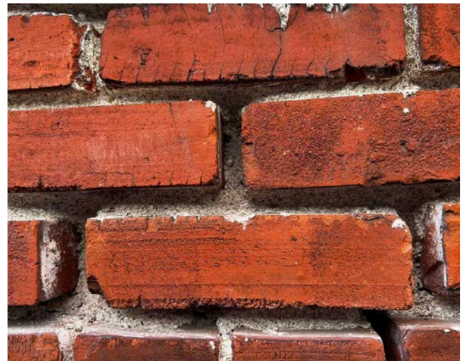
Figure 4.6 - Mortar is a sacrificial material that will deteriorate over time. It is important to check for areas in need of repointing before the structure of the building is compromised.
