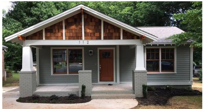
Figure 5.39 - The addition of a Craftsman style front porch (defined by the use of wood shingles, deep eaves, exposed rafter tails, and thick wood columns) to this Minimal Traditional style home is inappropriate.
