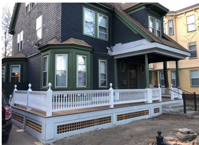
Figure 8.8 - Decks should not be constructed at the front of the building or attached to front porches, as shown above. It detracts from the historical features and creates a false sense of what the house historically looked like.
