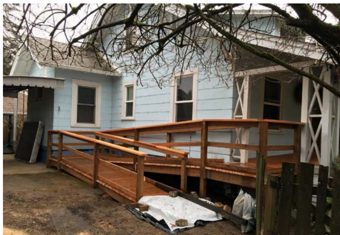
Figure 8.7 - This ADA ramp is sympathetic to the building's historical design. It is simple in design and material and placed along a secondary elevation with access to front porch from the side. If it is eventually removed, the balustrade can easily be replicated and reinserted.
