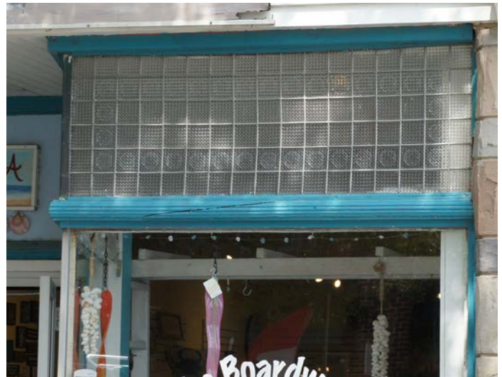
Figure 4.14 - Storefront transom windows, like the one shown above, are often painted over or covered by modern awnings that alter the historic storefront. These should be retained and repaired as necessary. If broken, a new glass pane should match the texture and size as the remaining historic panes.
