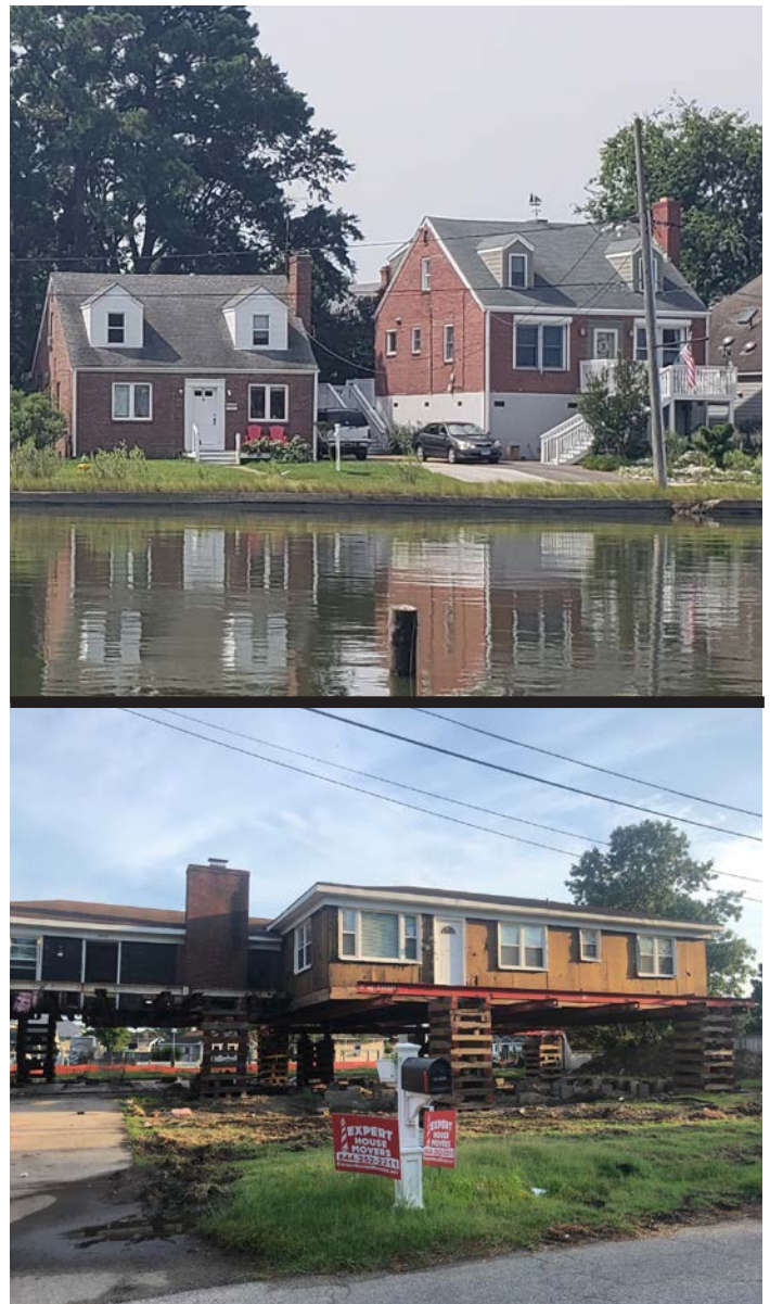
Figure 10.11 - Elevating a historic home significantly alters its appearance and historic materials (top photograph). It is also an extremely costly and delicate procedure and should be a last-resort measure for historic buildings (bottom photograph).
