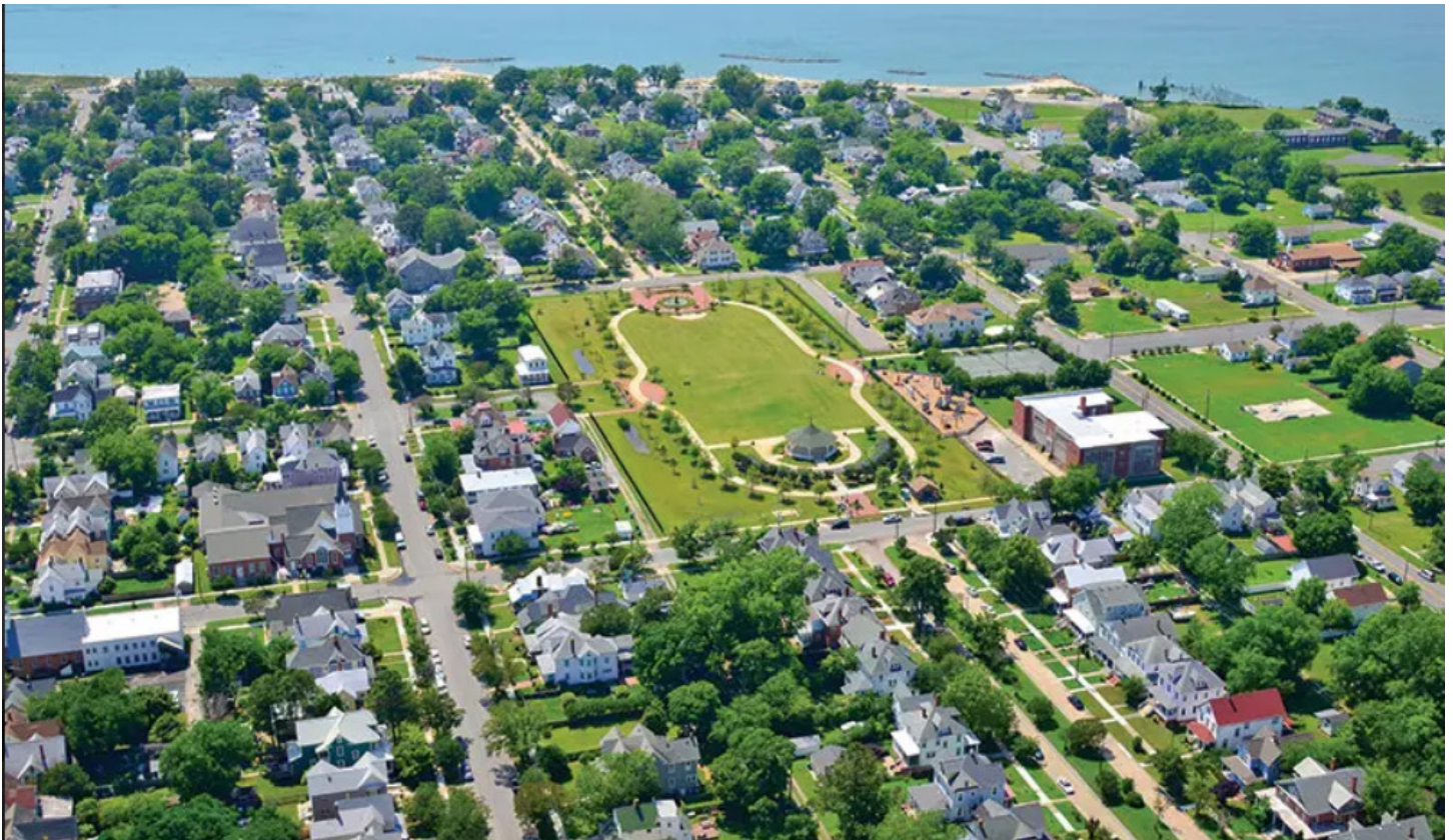
Figure 1.1 - A current aerial of the Cape Charles Historic District. (Photo by Chris Glennon)
