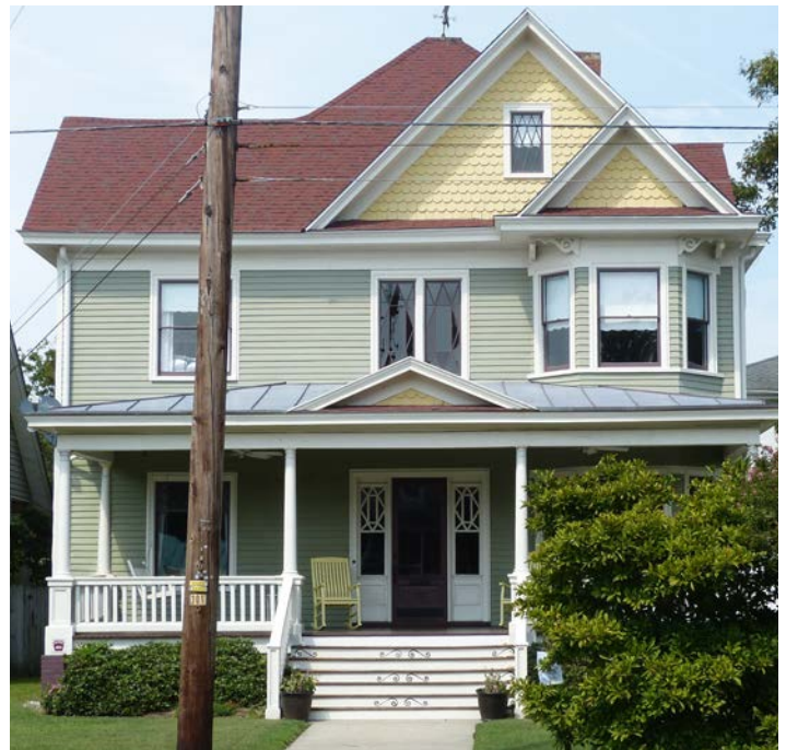
Figure 4.3 - Often porches or one-story protrusions will have metal roofs that are different from the main roof, like the standing seam metal porch roof shown above.
