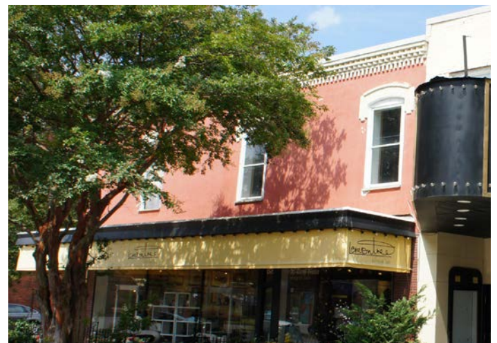
Figure 5.8 - Cape Charles has few examples of extensive stucco work. A rare example is shown above.
