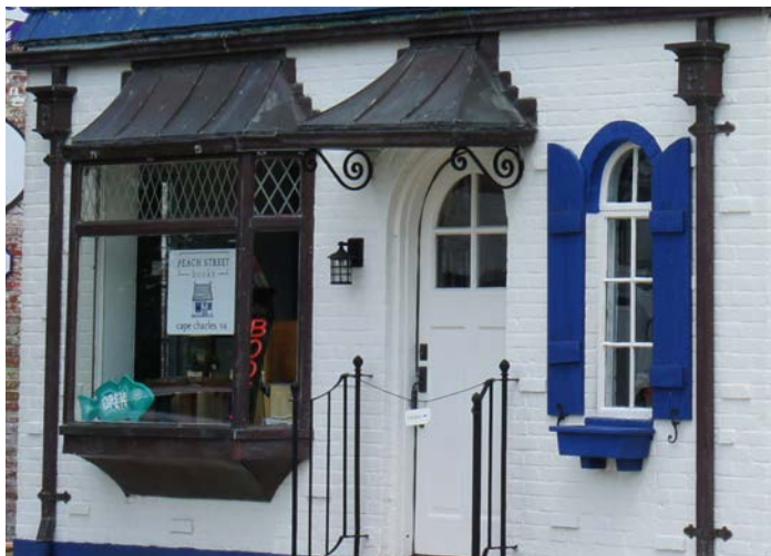
Figure 5.21 - Cape Charles has a wide variety of historic window designs and features, both to residential and commercial resources. These should be retained and maintained.
