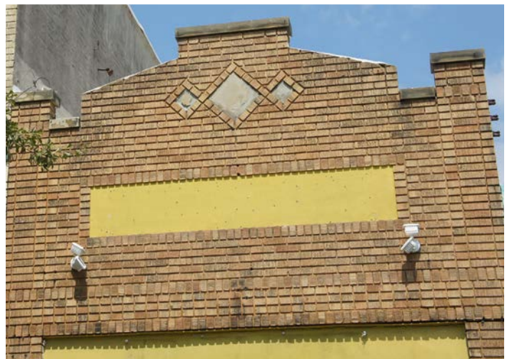
Figure 5.6 - The multiple brick designs on the residential and commercial facades above are character-defining features. They should be retained and remain uncovered.
