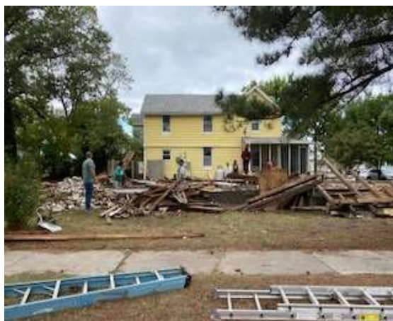
Lot Immediately after Demolition – 10/13/2021
