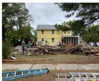
Lot Immediately after Demolition – 10/13/2021
