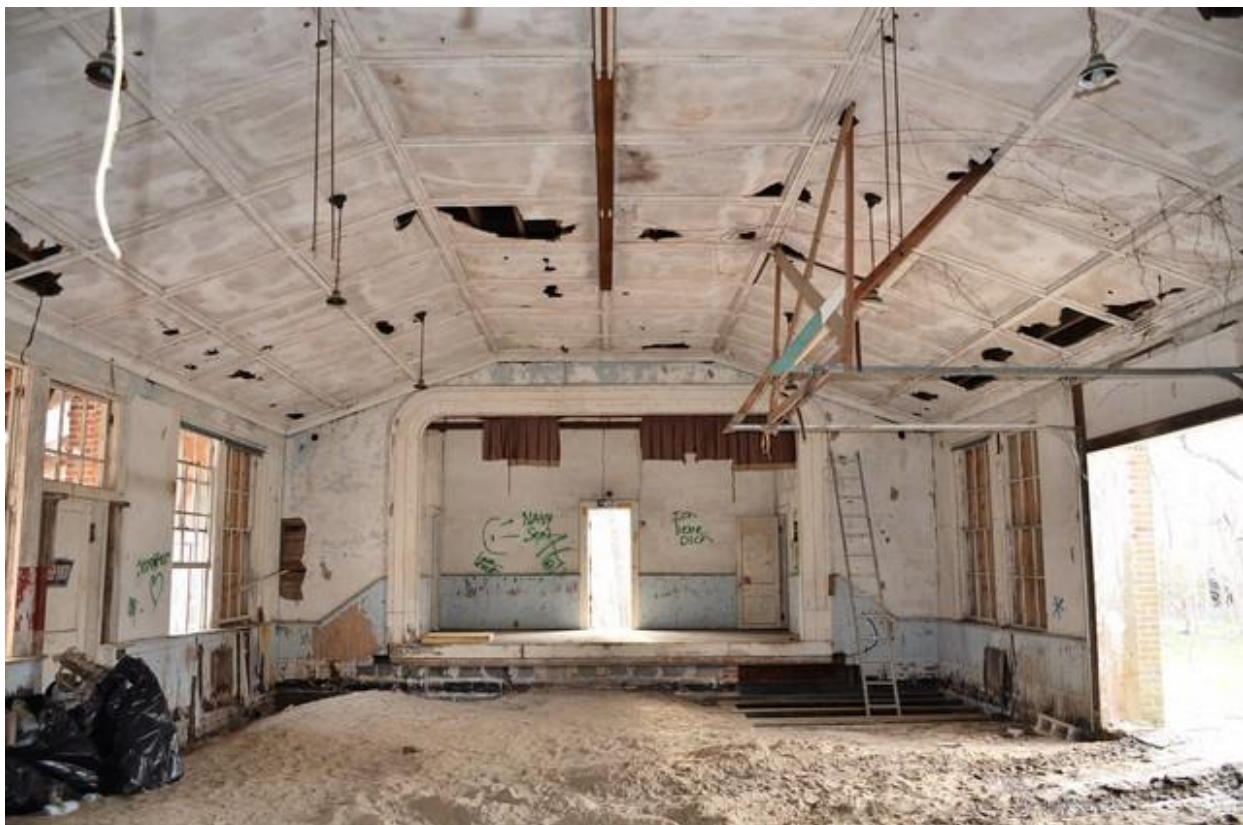
Cape Charles Elementary School – Interior View of the Auditorium Facing West (Courtesy of The Patina Group)
