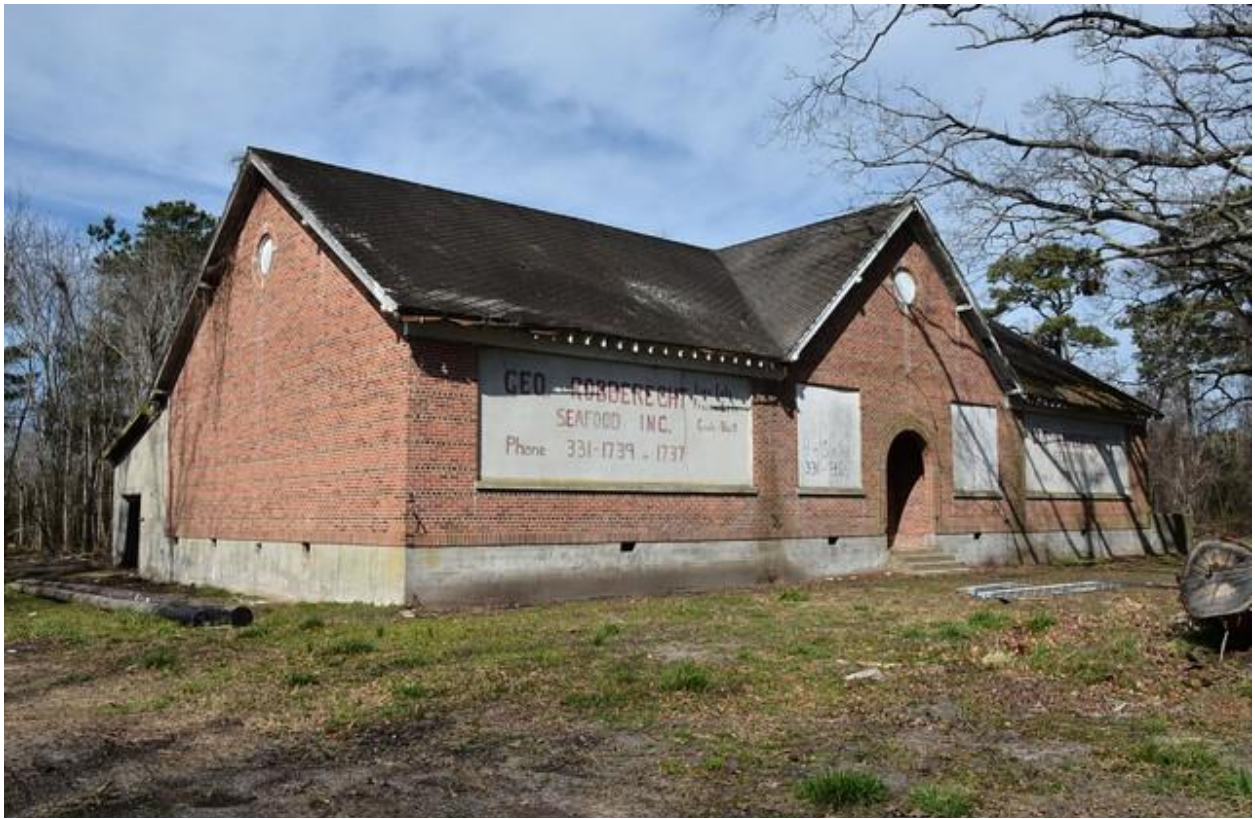
Cape Charles Elementary School - View from the Southeast (Courtesy of The Patina Group)
