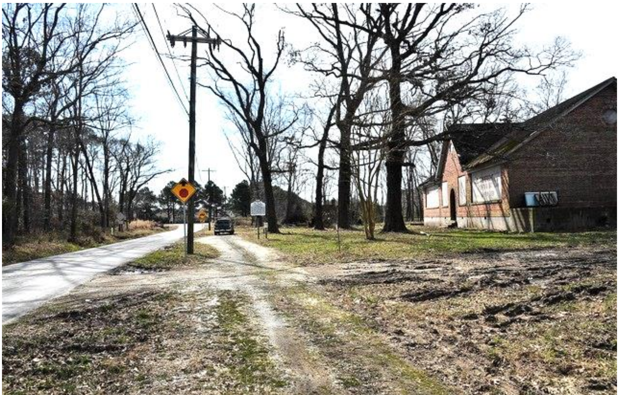
Cape Charles Elementary School - View from the North (Courtesy of The Patina Group)
