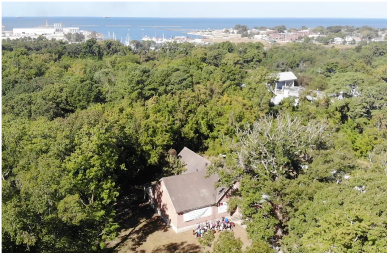
Cape Charles Elementary School – Aerial View from the East (Courtesy of Dr. M. Potter Henderson)
