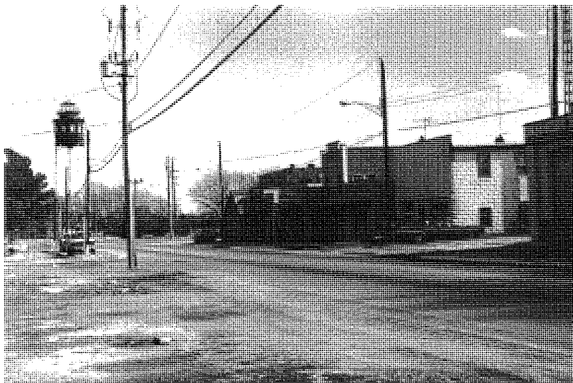
Plate No. 4. Route 184 at the entrance to Cape Charles lacks the character and definition that could be provided by appropriate landscaping.
