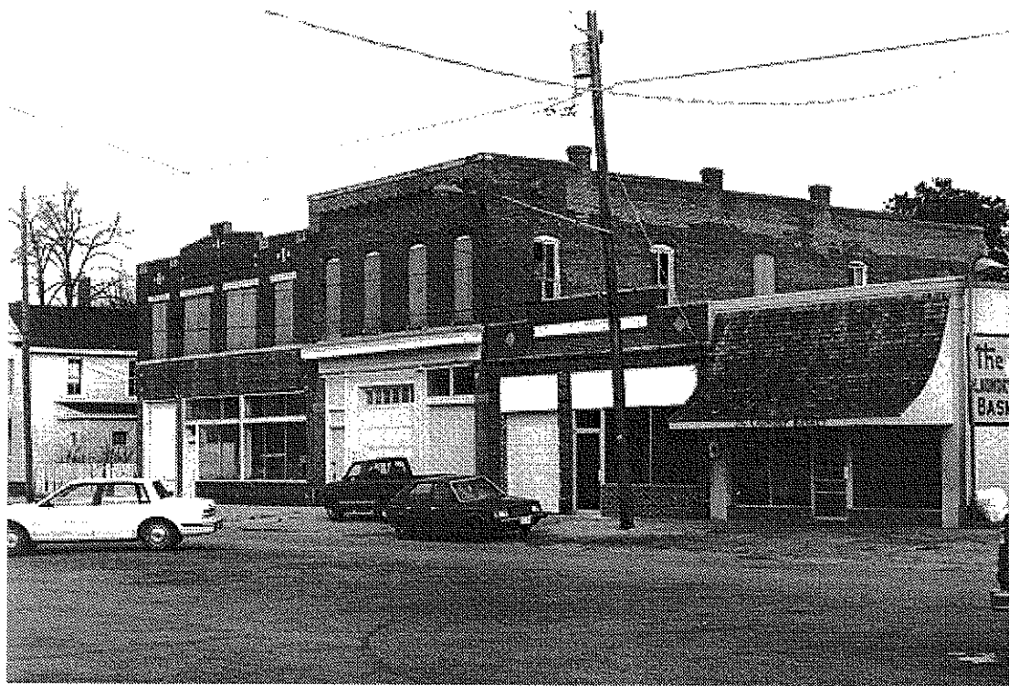
Plate No. 14. Underutilized and vacant commercial buildings on Peach Street.
