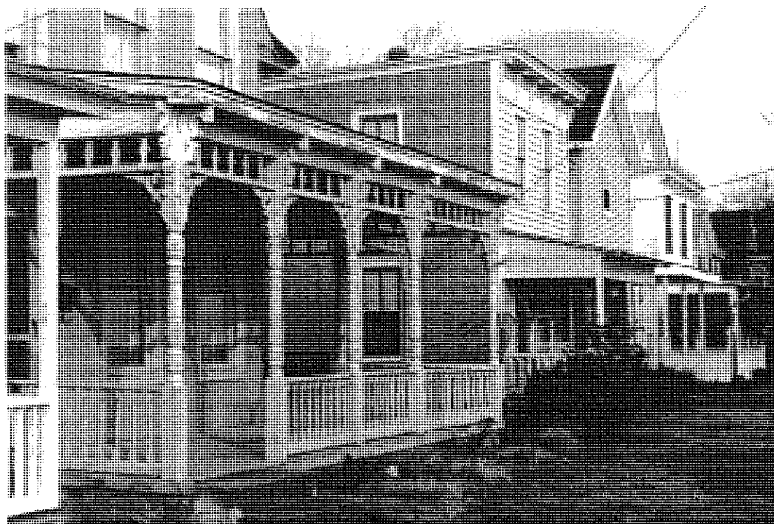
Plate No. 31. The town's many porches should be preserved through proper maintenance.
