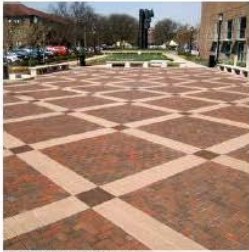
Cross Pattern Brick Paving
