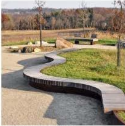
Seat walls with wooden planks
