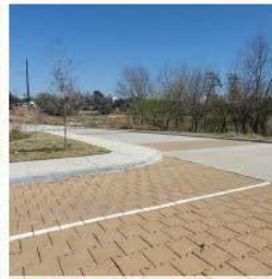
Pavers used for parking bays
