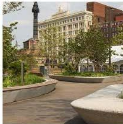
Cast in place concrete seat walls
