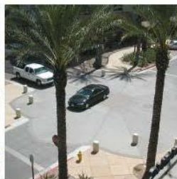
Curbless intersection with protective bollards
