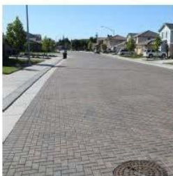
Pavers used for roadways
