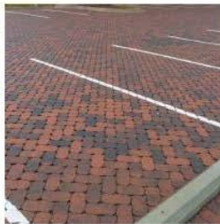
Permeable brick paving
